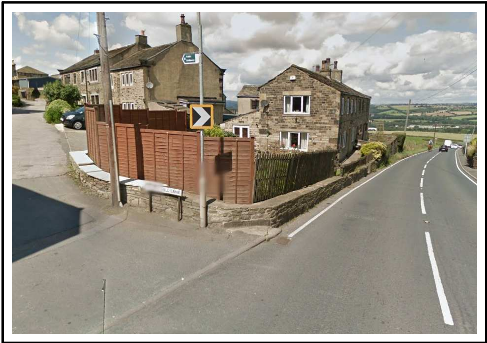
Picture of dissimilar fencing prior to wind damage to east boundary fence
