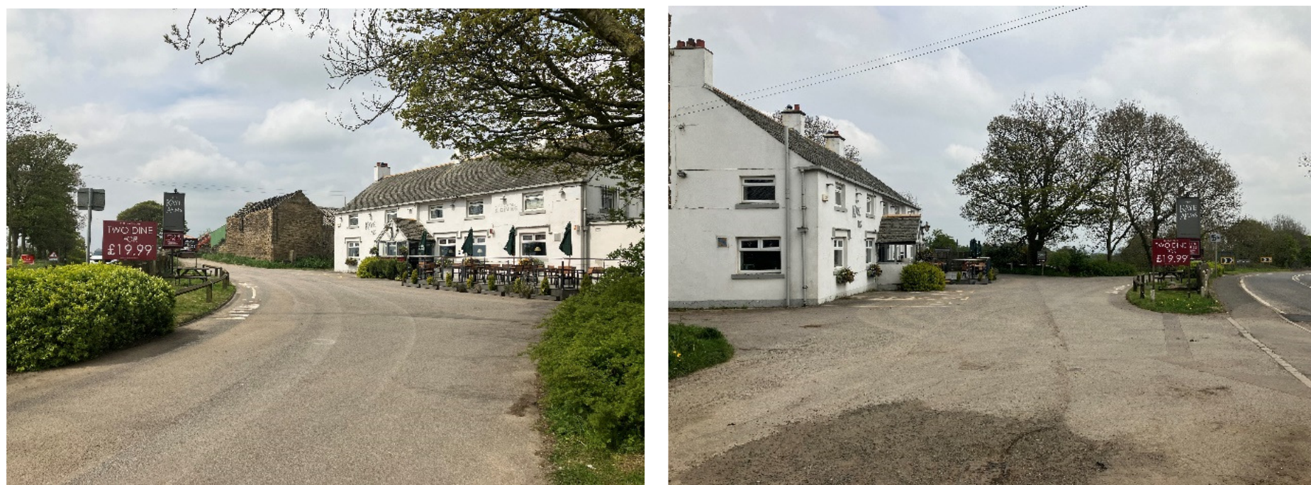
General View - Existing Front (South) Elevation to Wakefield Road
