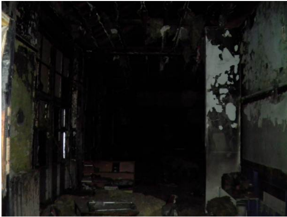
Photo 5 Overall view of main fire damaged rooms
