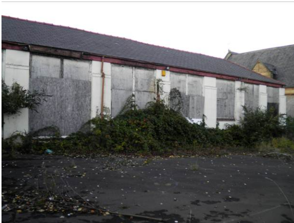
Photo 1 Overall view of eastern elevation
