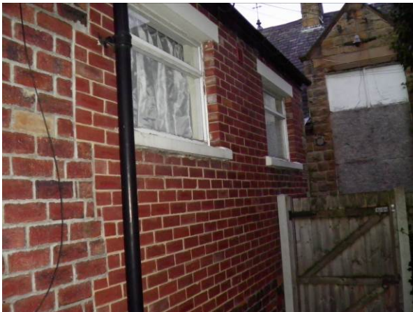
Photo 3 Extensions to rear elevation
