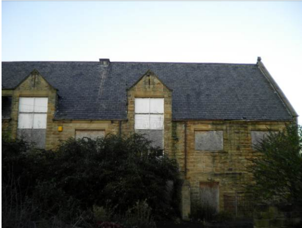
Photo 1 Typical view of side elevation
