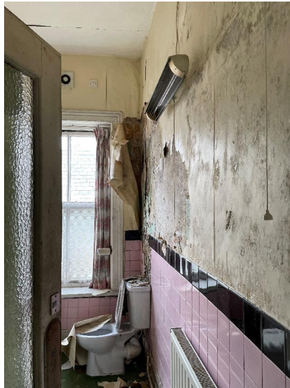
FF toilet damage due to water ingress
