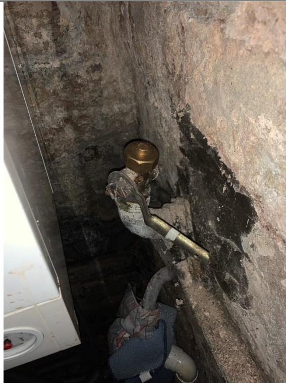
Gas meter removed
