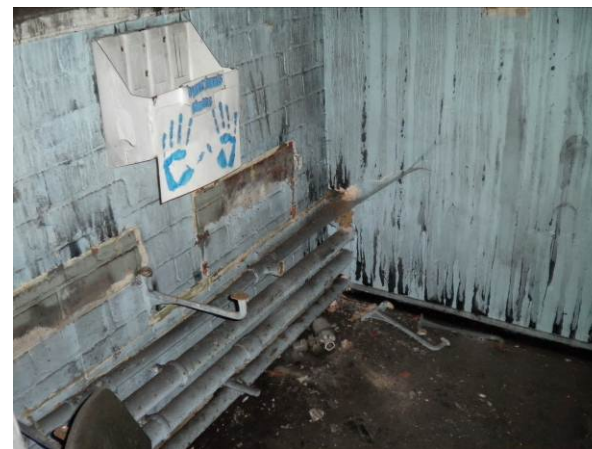
Photo 10 Typical view of toilet accommodation
