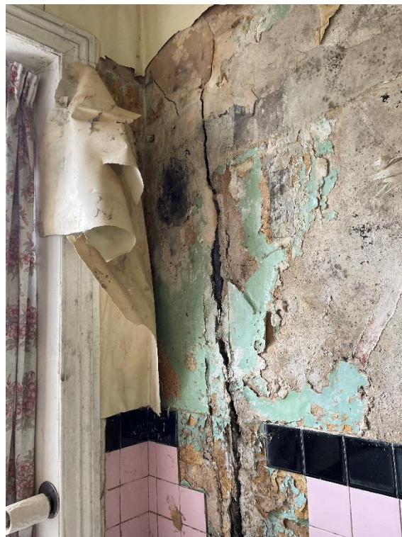
FF toilet damage due to water ingress
