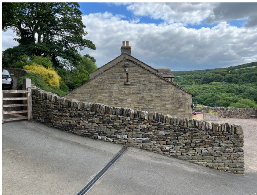
Fig.20 Photo of West Elevation from driveway
