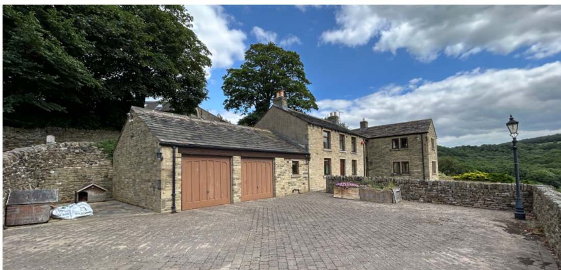
Fig4. View East from drive
