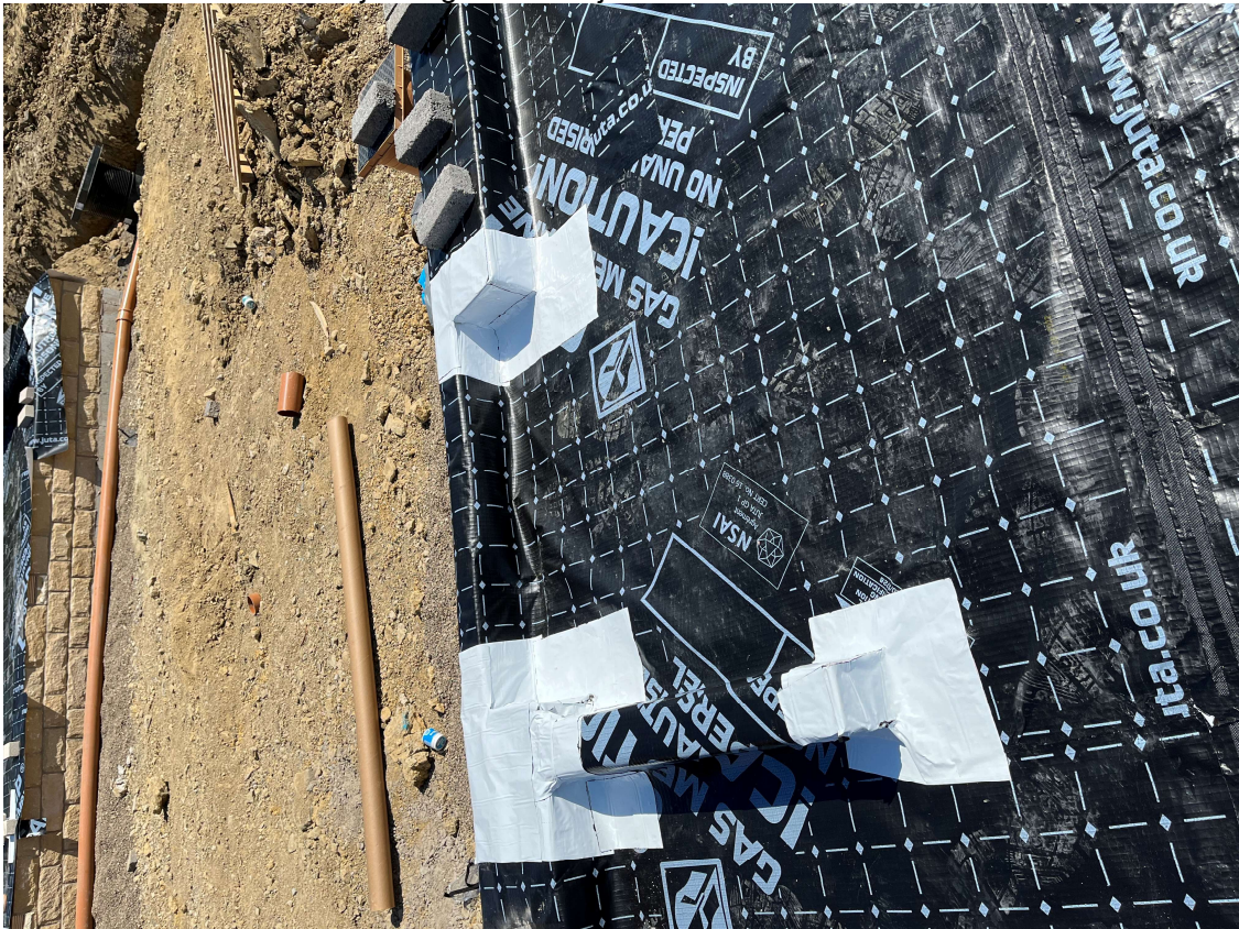
Plot 189 – Membrane and jointing with weld joint
