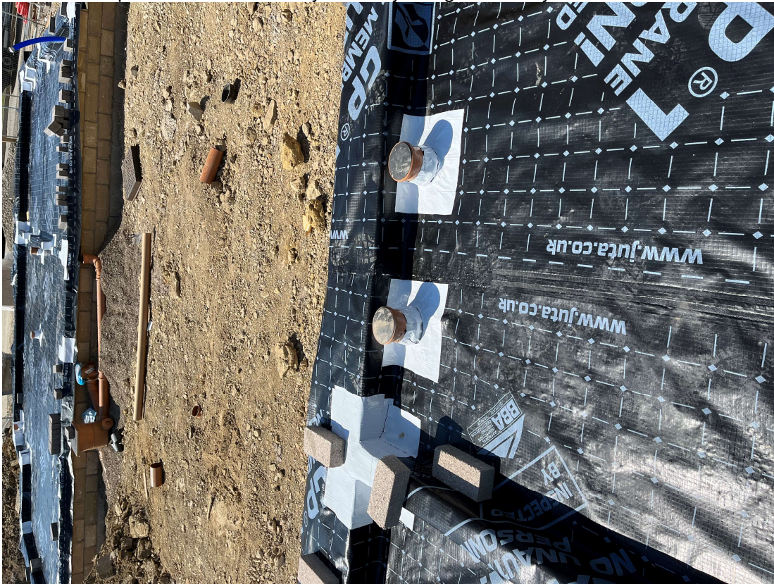
Plot 188 – Tophat and membrane layout with jointing and weld joint
