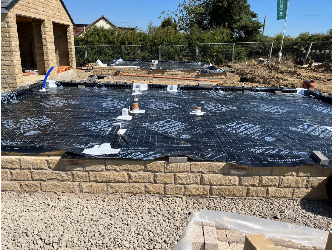
Plot 189 – Membrane and jointing with weld joint
