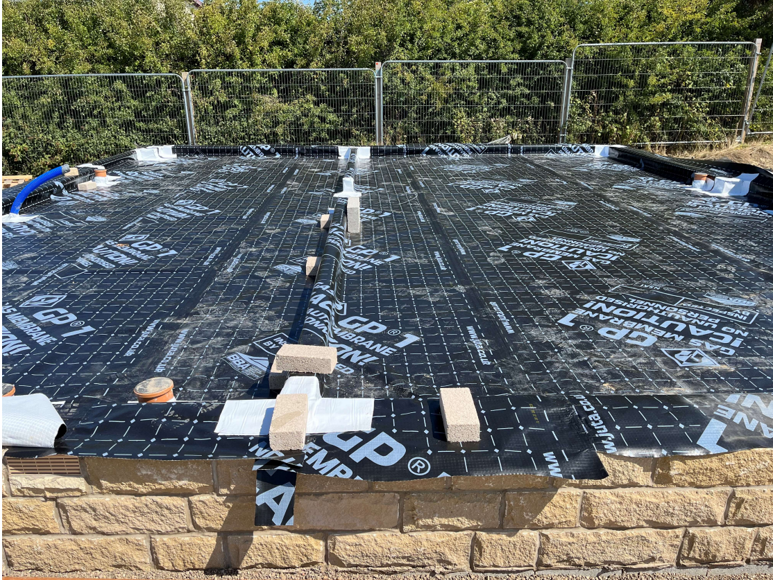
Plot 188 – Tophat and membrane layout with jointing and weld joint
