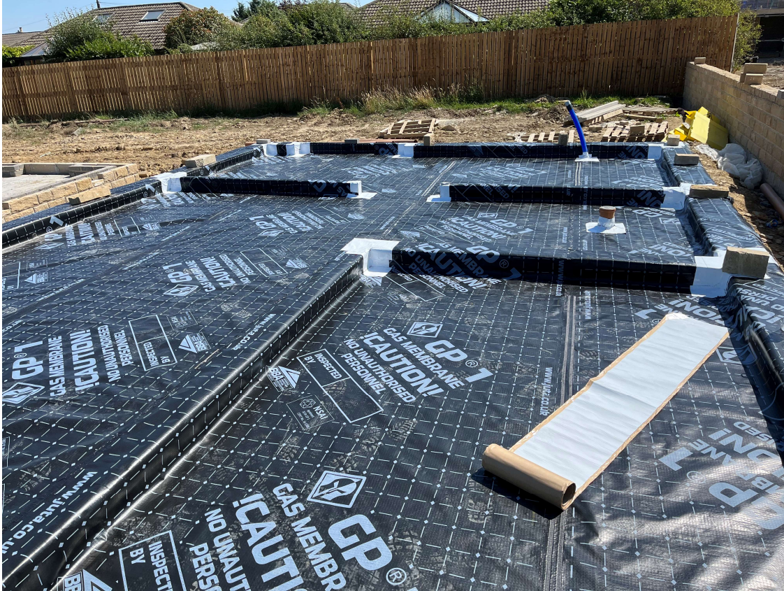
Plot 165 – Membrane layout with jointing
