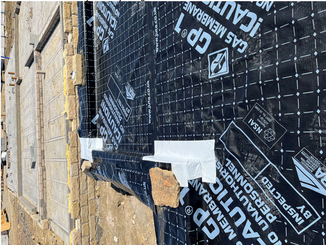
Plot 165 – Membrane layout with jointing
