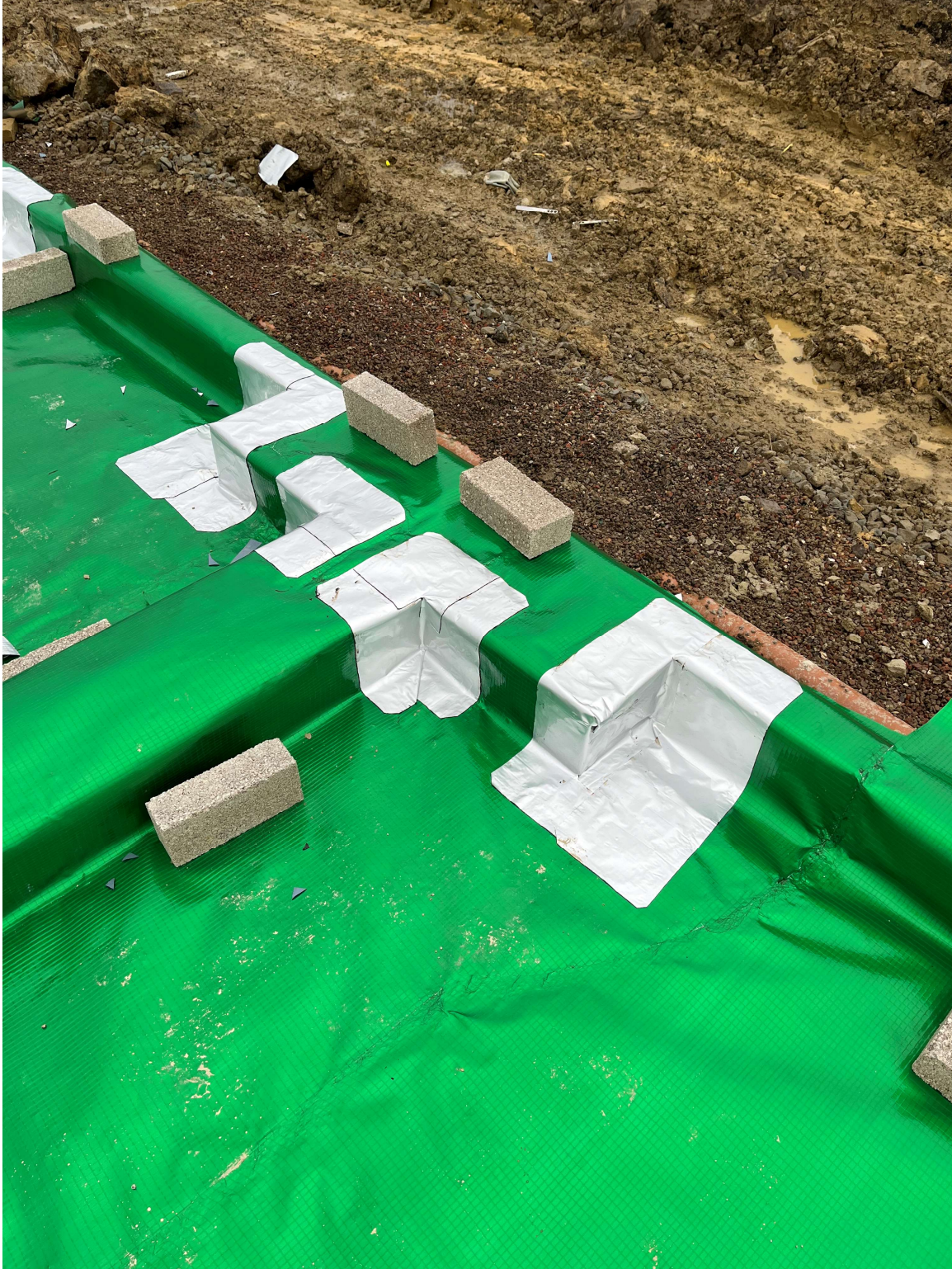
Plot 22 & 23 – membrane layout and jointing
