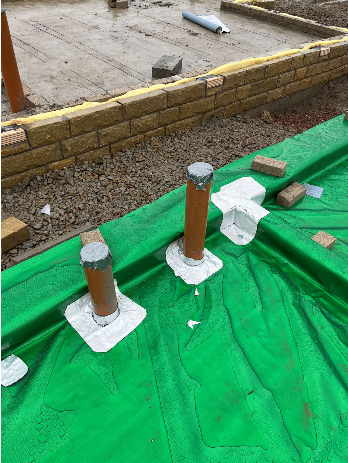
Plot 17 - Tophat & membrane layout and jointing
