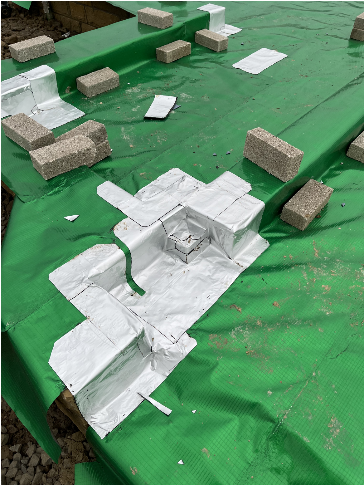
Plot 20 - membrane layout and jointing
