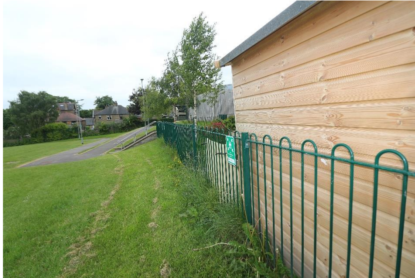
Image 5: Current bow tie fencing to rear
