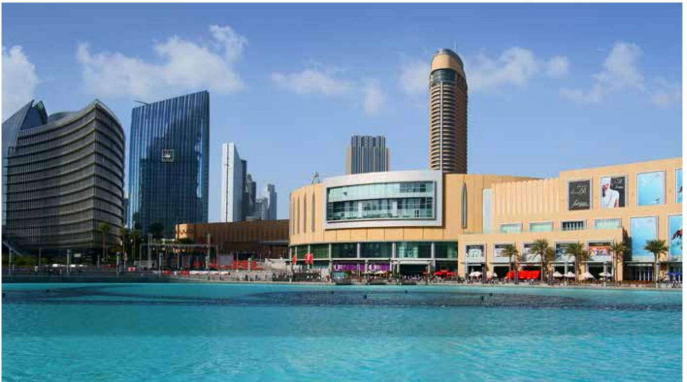
Dubai Mall - Purified Air provided filtration for the food & beverage outlets
