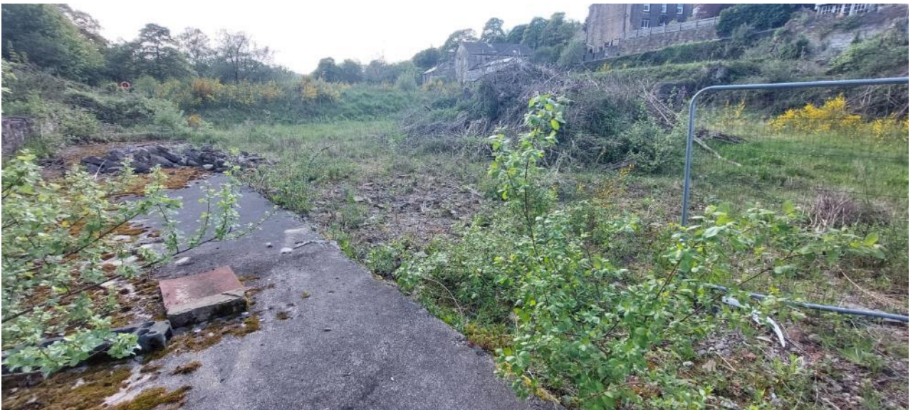
Image 2: Areas of hardstanding within the site
