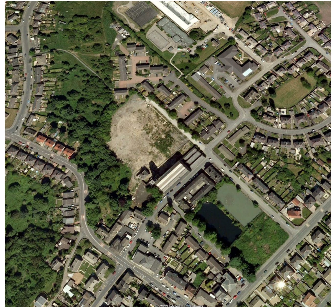
Google Earth Aerial Photo 2009 – site has largely been cleared other than the main mill structure on Ruth Street.
