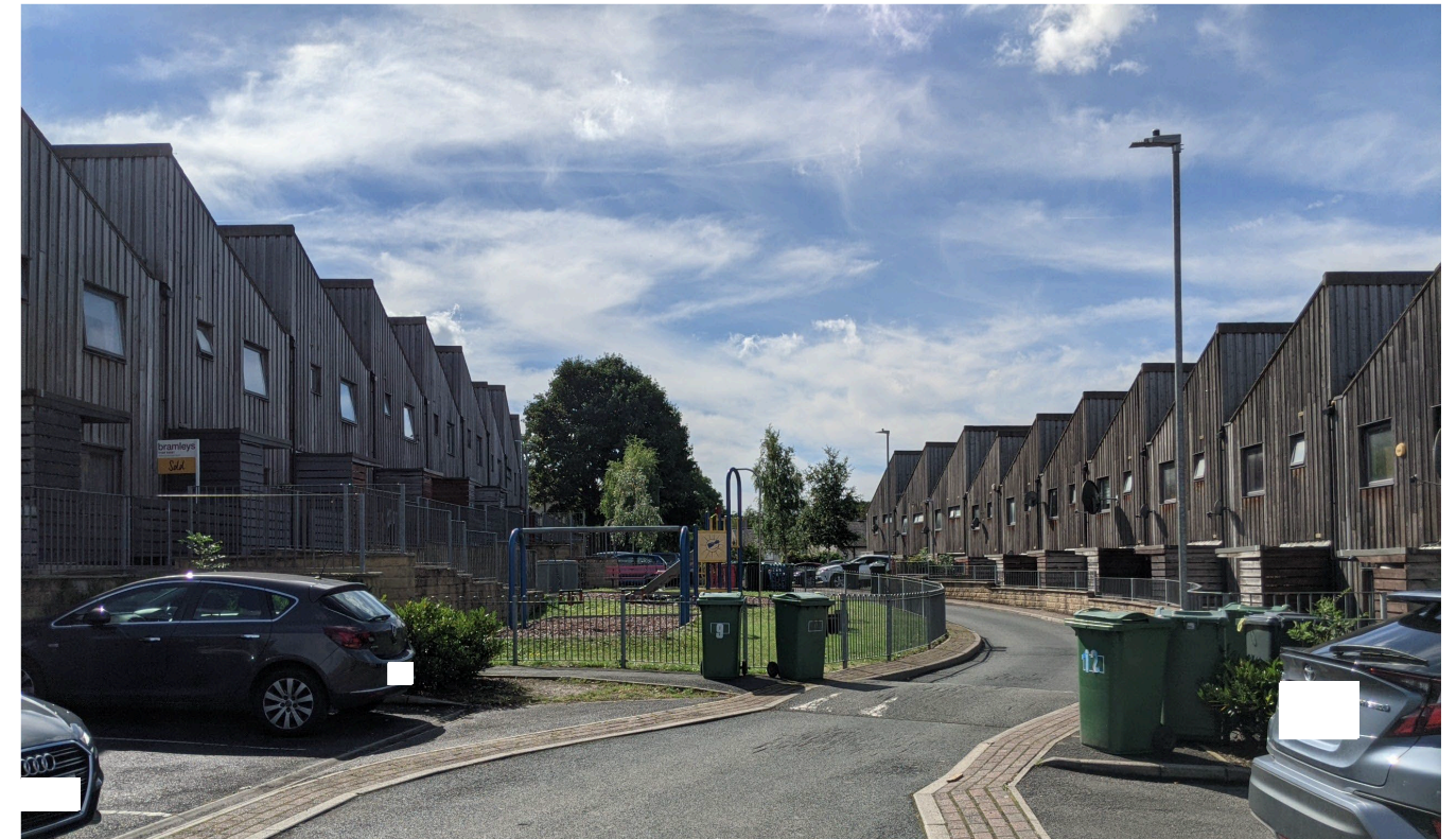
Contemporary 2-storey timber-clad houses in Ridge Street, with sawtooth roof mimicking historic Newsome Mill
