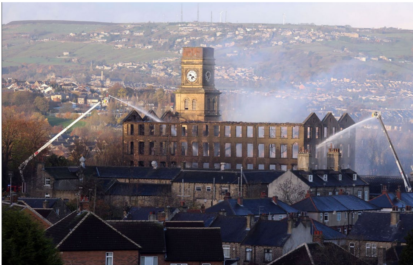
November 2016 Photograph – a devastating fire gutted the grade II listed structure and the roof/ floors collapsed. The building was deemed unsafe and brought down to its current first floor level. Credit: Yorkshire Live
