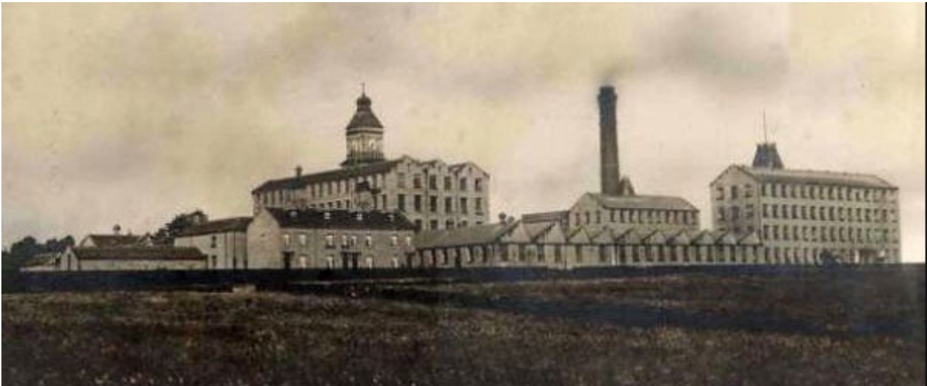
Composite Photo – date unknown but assumed between 1916 and 1932 based on comparison between Ordnance survey maps. Image was likely prior to aerial photo as clock tower roof is tapered. Credit – HughieDW [Flickr]
