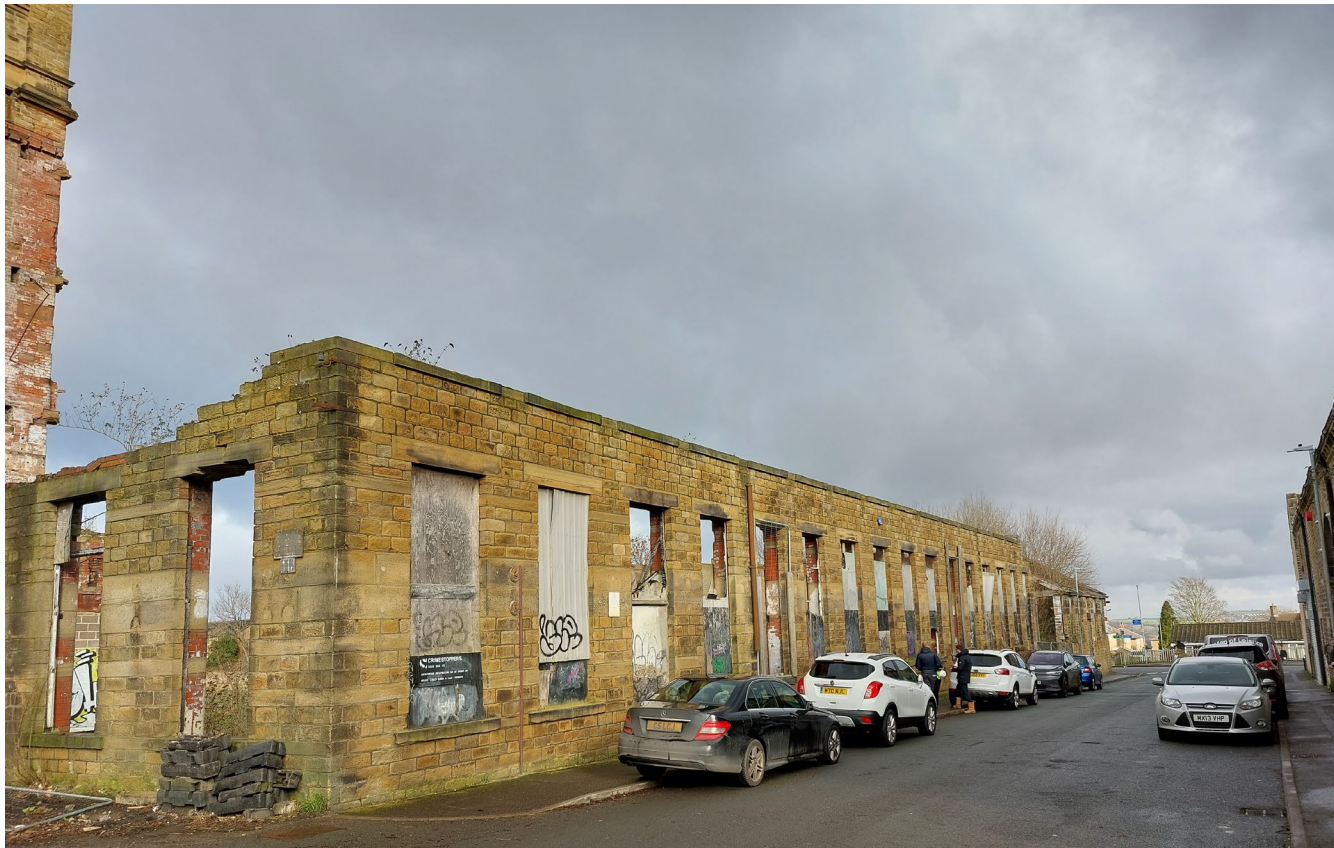
Site Photos of Newsome Mill remains taken 27 th January 2023.
