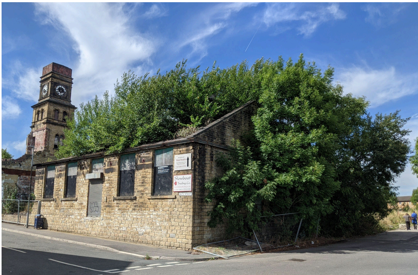
Site Photo of Weaver Sheds taken 5 th September 2022.
