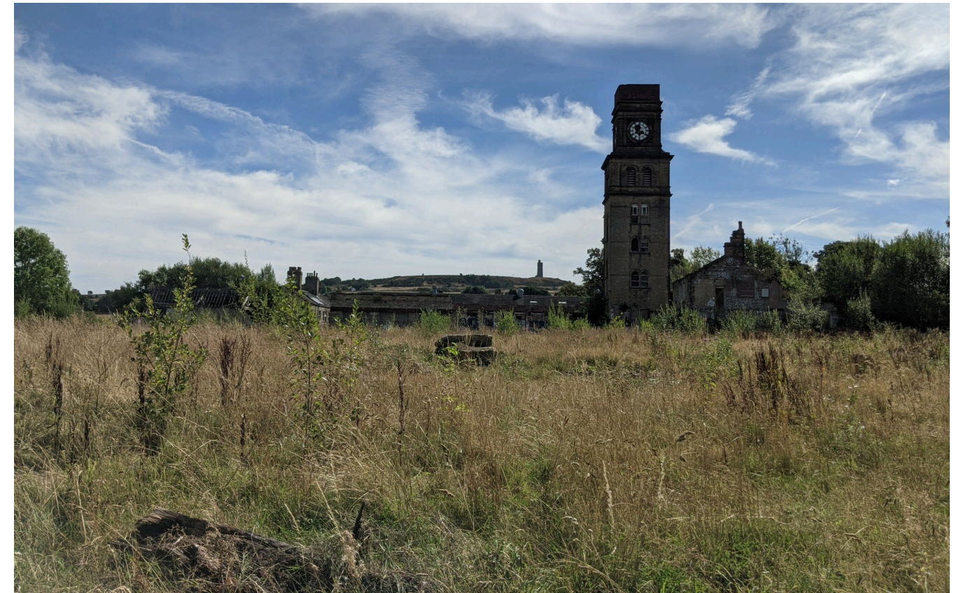
Site Photos of overgrown rear site taken 5 th September 2022.
