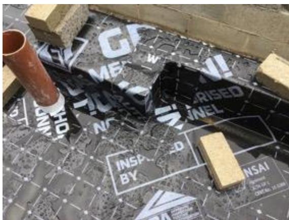
Plot 8p pipe penetration sealed using preformed top hat and SAGM and door threshold using preformed corners
