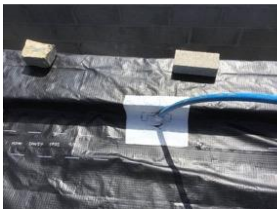
Plot 10 corner detail using preformed corners
