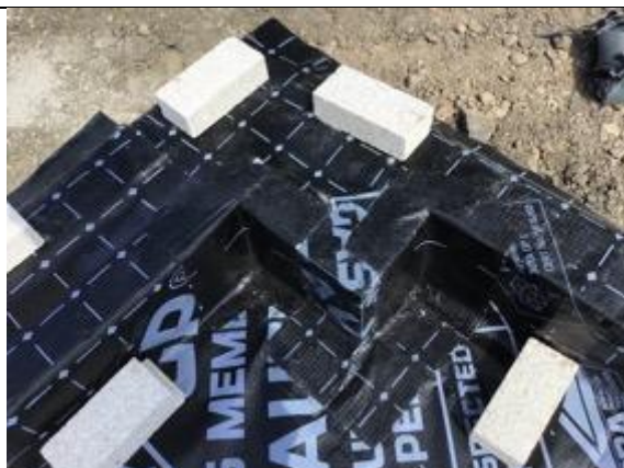
Plot 10 corner detail using preformed corners
