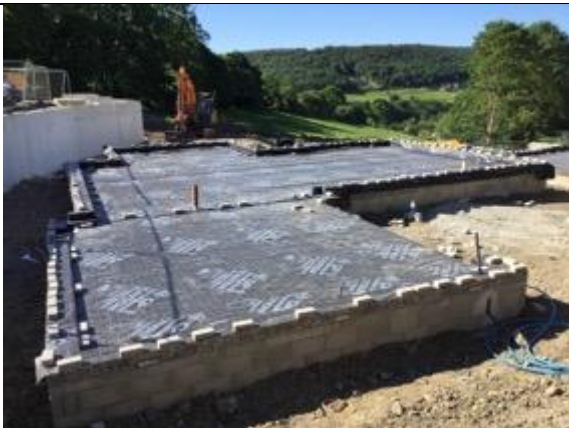
Overview photo looking at Plot 4"
