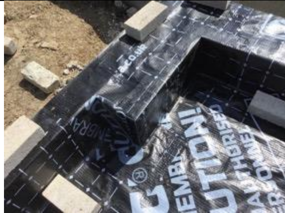
Plot 11 door threshold and corner detail using preformed corners
