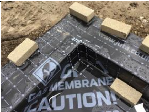
Plot 7 corner detail using preformed corners
