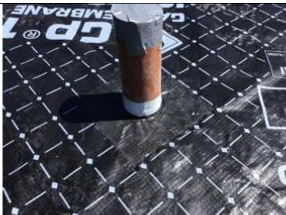
Plot 6 sealed pre formed pipe penetration top hat
