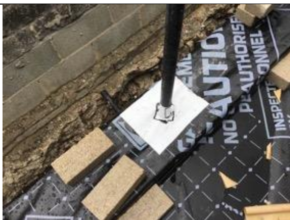
Plot 8 service pipe seal using SAGM
