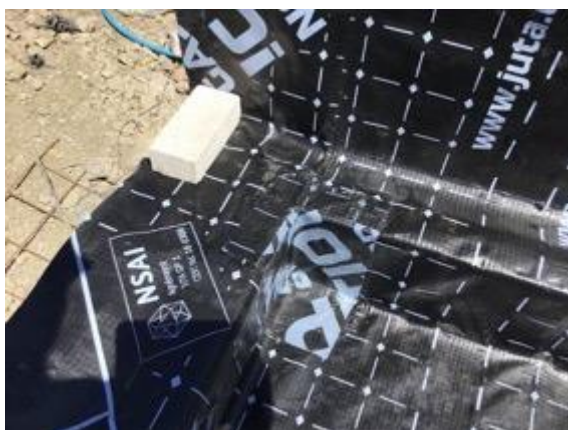
Plot 6 sealed pre formed pipe penetration top hat
