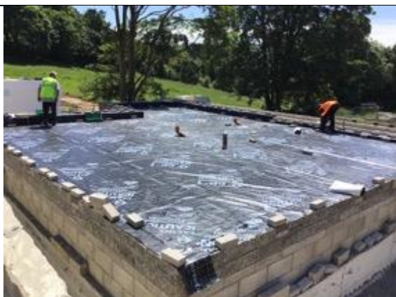
Plot 9 full line out installation
