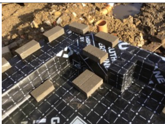
Plot 16 corner detail and door threshold using preformed corners
