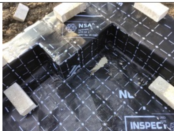
Plot 17 corner detail and door threshold using preformed corners
