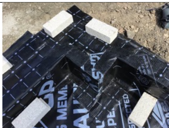
Plot 10 corner detail using preformed corners
