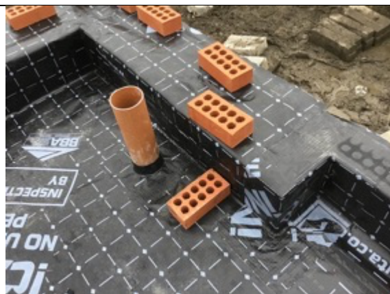
Plot 13 door threshold and corner detail using preformed corners and pipe penetration sealed using preformed top hat and SAM
