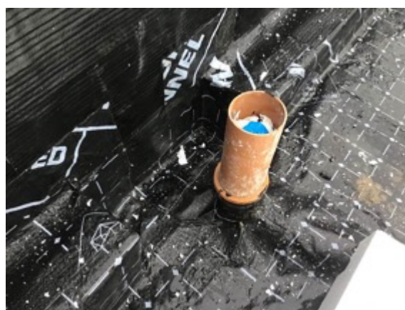
Plot 3 sealed pipe penetration
