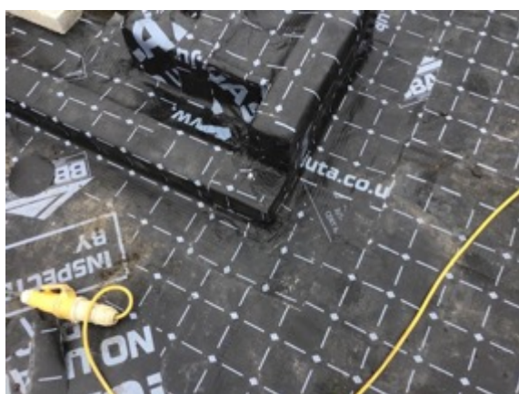
Plot 12 detailing using preformed corners
