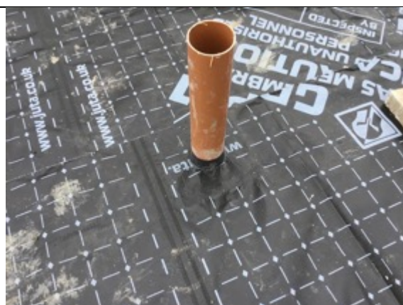
Plot 12 pipe penetration sealed using preformed top hat and SAM
