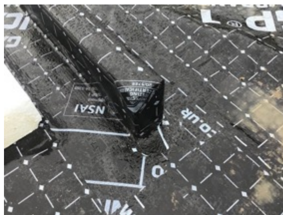
Plot 2 internal wall corner detailing
