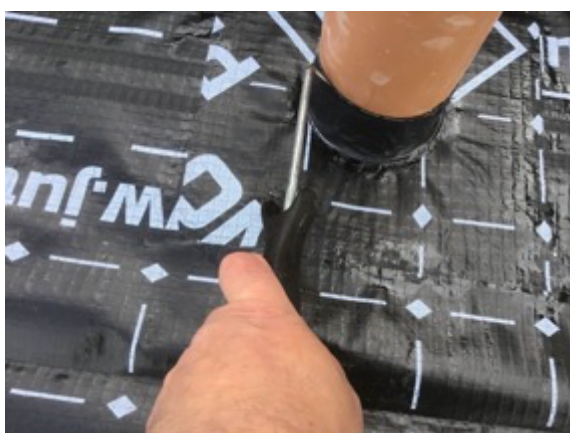
Pipe penetration sealed using preformed top hat and SAM being pick tested
