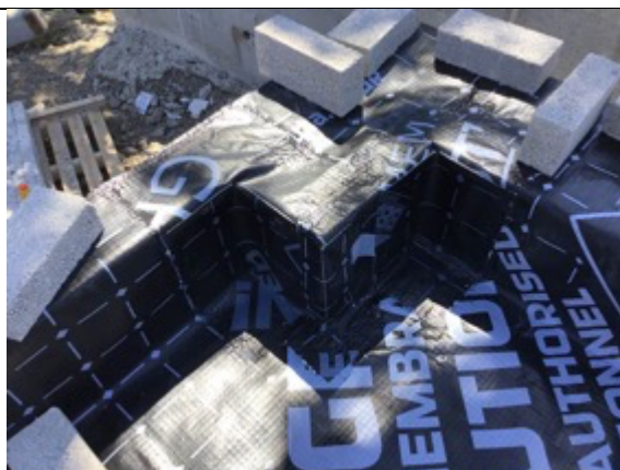
Plot 9 sealed pre formed corner and threshold detailing
