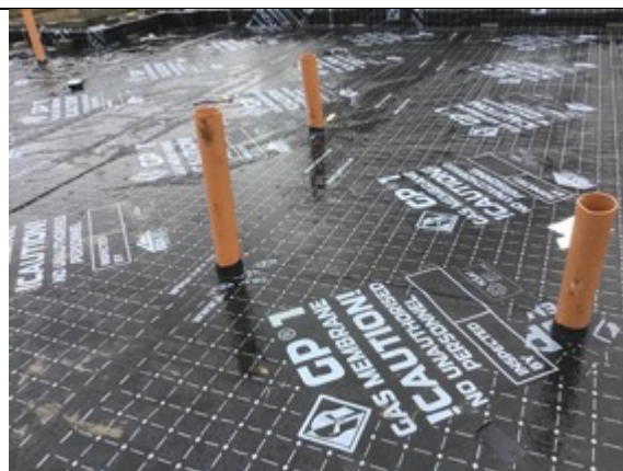
Plot 17 pipe penetrations sealed using preformed top hats and SAM
