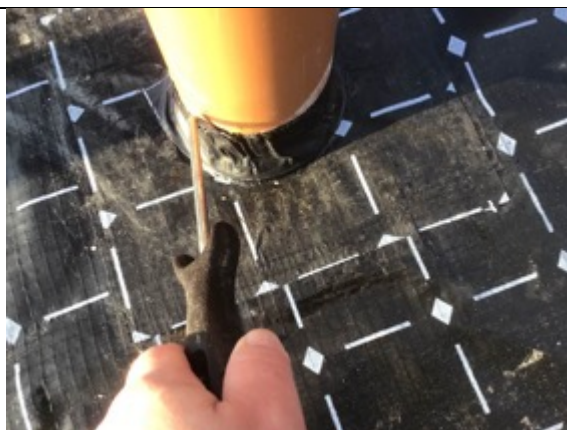
Plot 18 pipe penetration sealed using preformed top hat and SAM being pick tested
