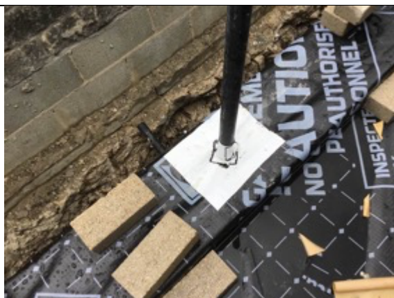
Plot 8 service pipe seal using SAGM
