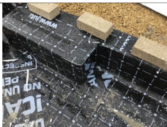
Plot 3 sealed threshold detail
