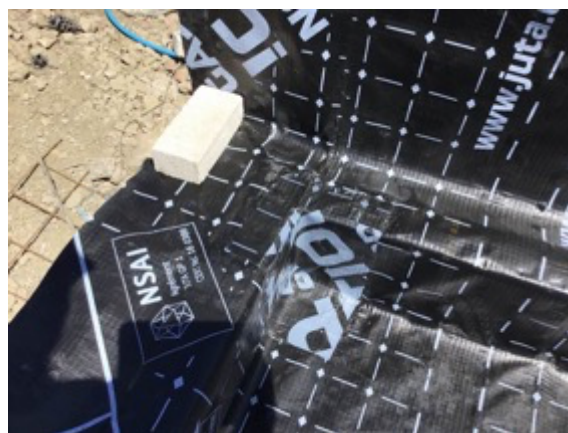
Plot 6 sealed pre formed pipe penetration top hat
