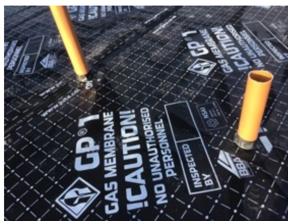
Plot 17 pipe penetrations sealed using preformed top hats and SAM
