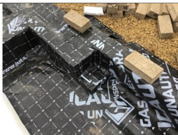
Plot 2 sealed threshold detail
