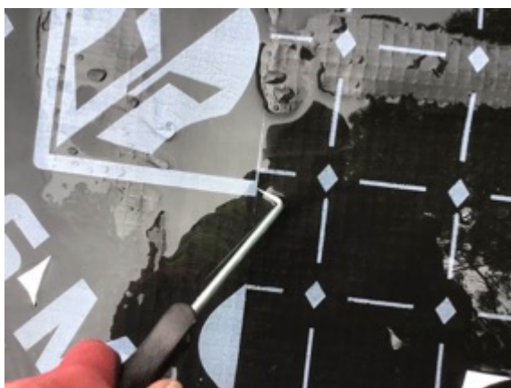
Plot 8 hand welded joint being pick tested
