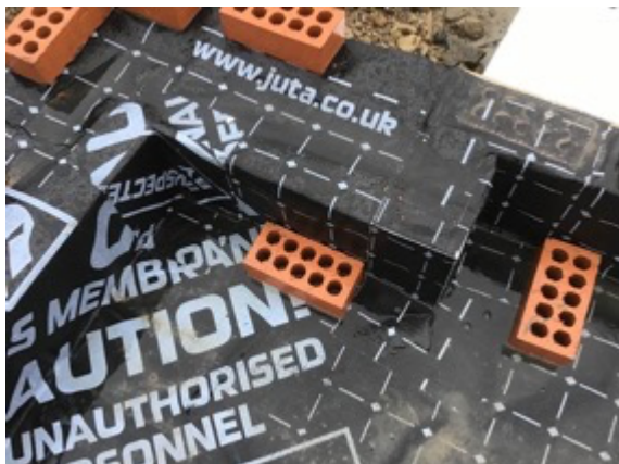
Plot 14 corner detail and door threshold using preformed corners
