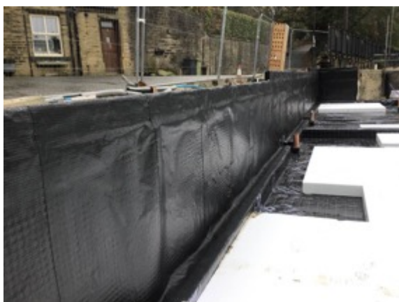
Retaining wall tanking detail
