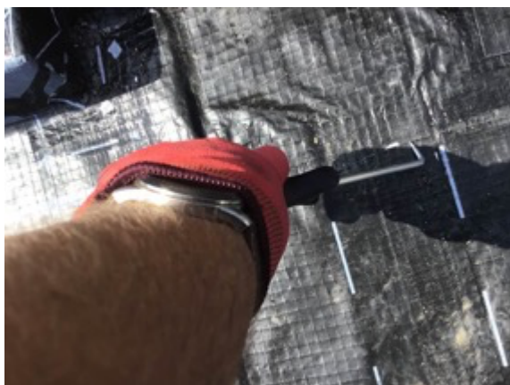
Plot 11 hand welded joint being pick tested
