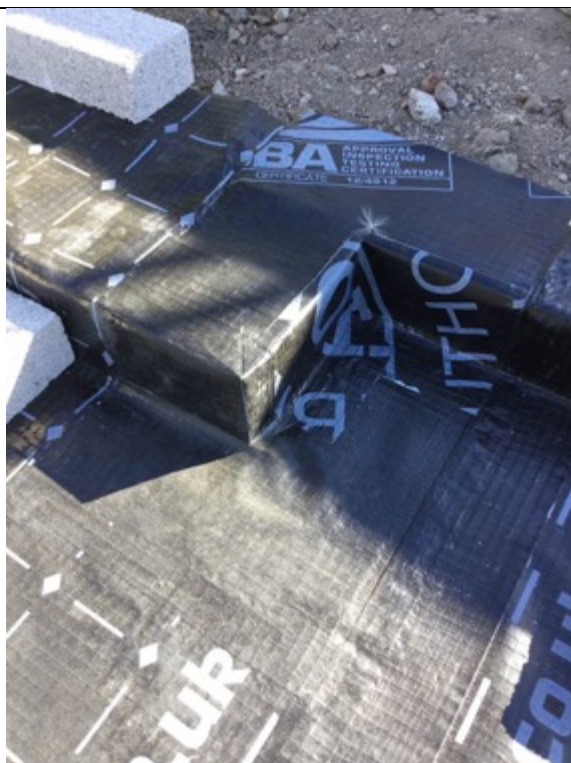
Close up showing the pre formed corner details for this doorway threshold.
