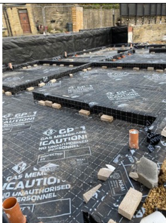
Plots 3 & 2 full line out installation
