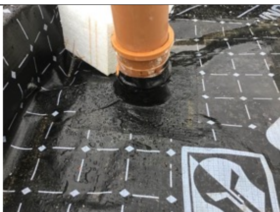
Plot 2 sealed pipe penetration
