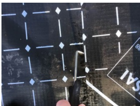
Plot 17 hand welded joint being pick tested
