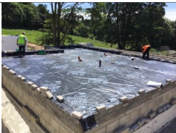
Plot 9 full line out installation
