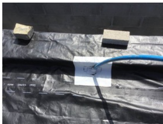
Plot 10 corner detail using preformed corners
