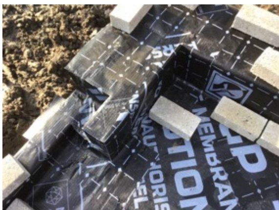
Plot 18 corner detail and door threshold using preformed corners
