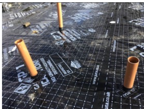
Plot 16 pipe penetrations sealed using preformed top hats and SAM
