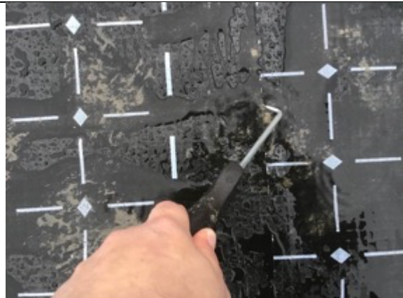
Plot 14 hand welded joint being pick tested
