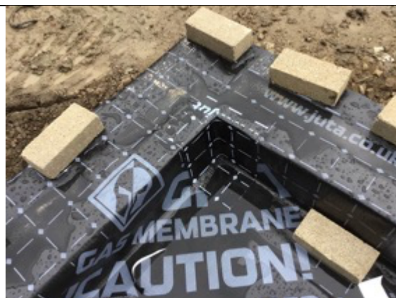
Plot 7 corner detail using preformed corners
