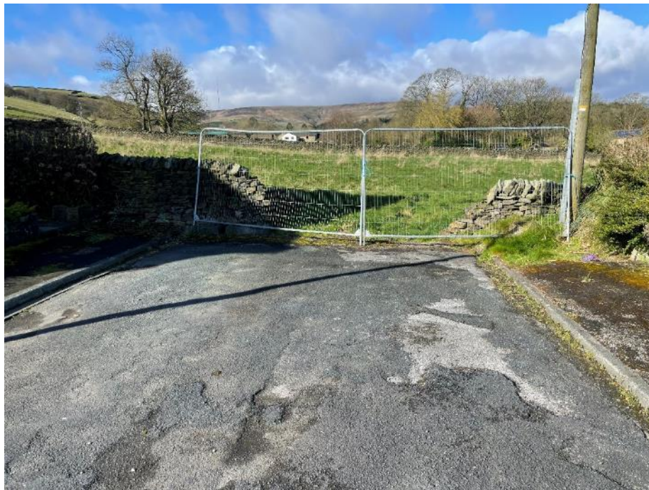
Photograph 2 – View of existing surfacing on Bankfield Drive
