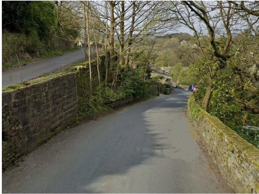
Photograph 4 – View of missing sign location in 2023 on Smithy Lane
