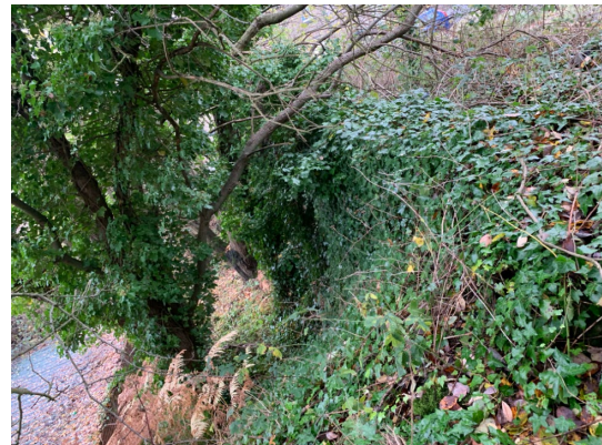
Photograph 8 – Built linear features, mortared wall featuring overhanging dense ivy.
