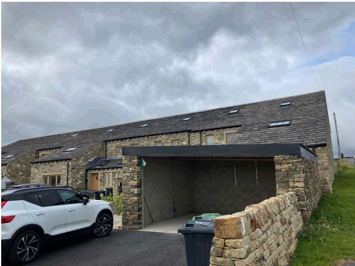
Photograph 2 - The rebuilt outbuilding. Although re-orientated please note open frontage, stone walls and cladding roof.
