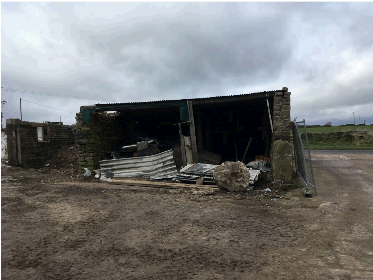
Photograph 1 - Outbuilding prior to development commencing. Note open frontage, stone walls and corrugated roof.
