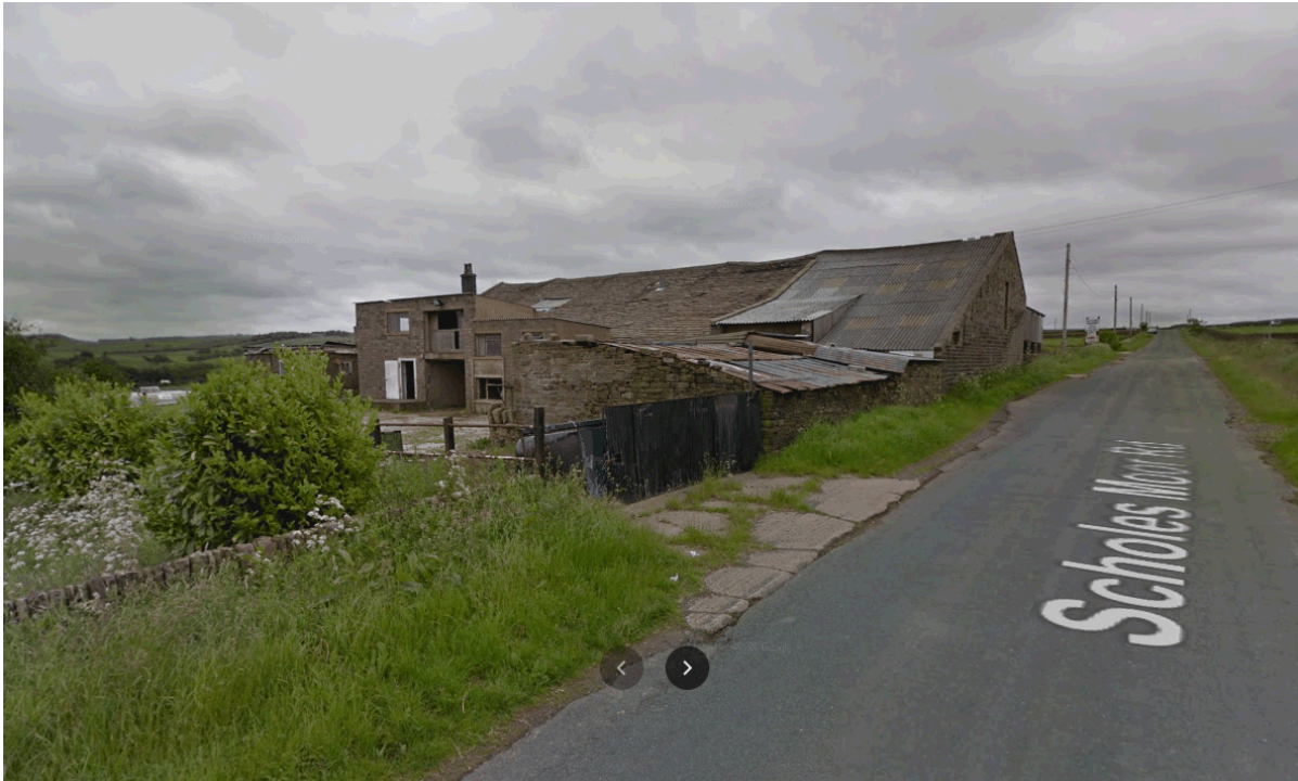
Image 3 - The original outbuilding prior to development work commencing.
