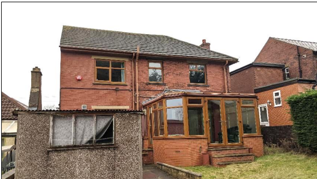
Plate 1. Rear (southwest) elevation of dwelling, with detached garage in foreground on left of image
