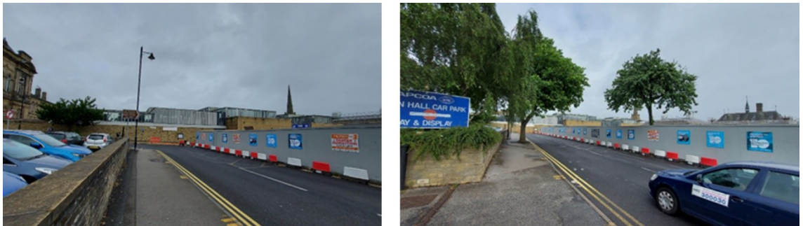
Plate 54: Views of the spire from the southwest and across the former car park site.
