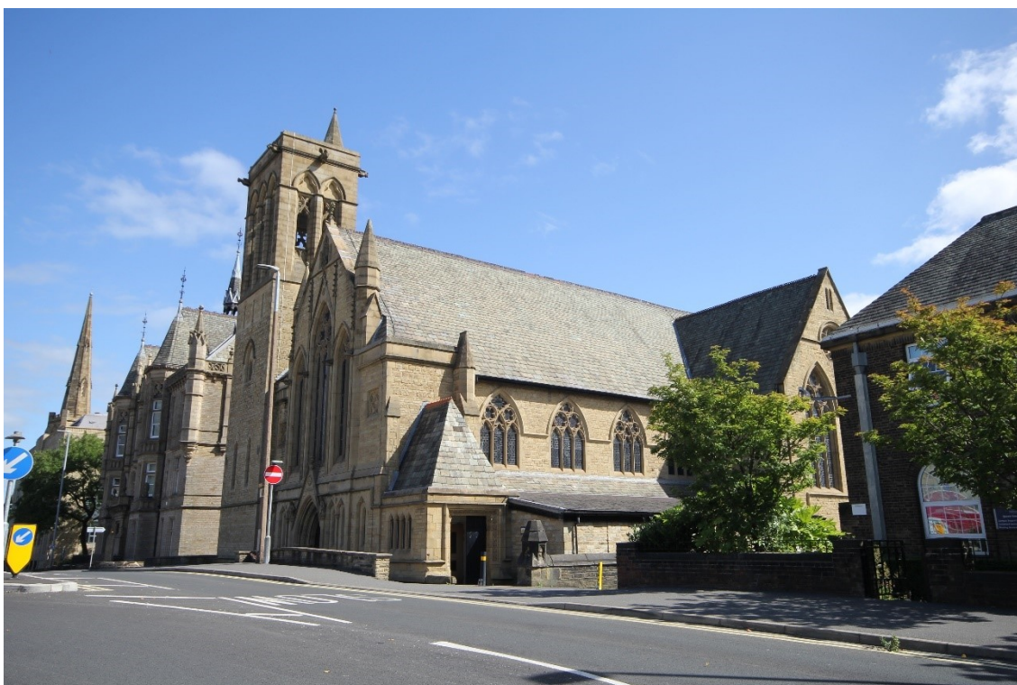
Plate 61: Milton Congregational Church
