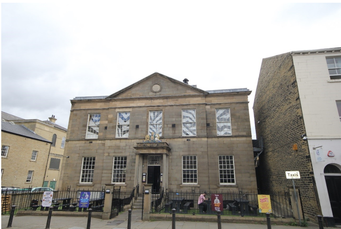
Plate 51: The Crown Court building.
