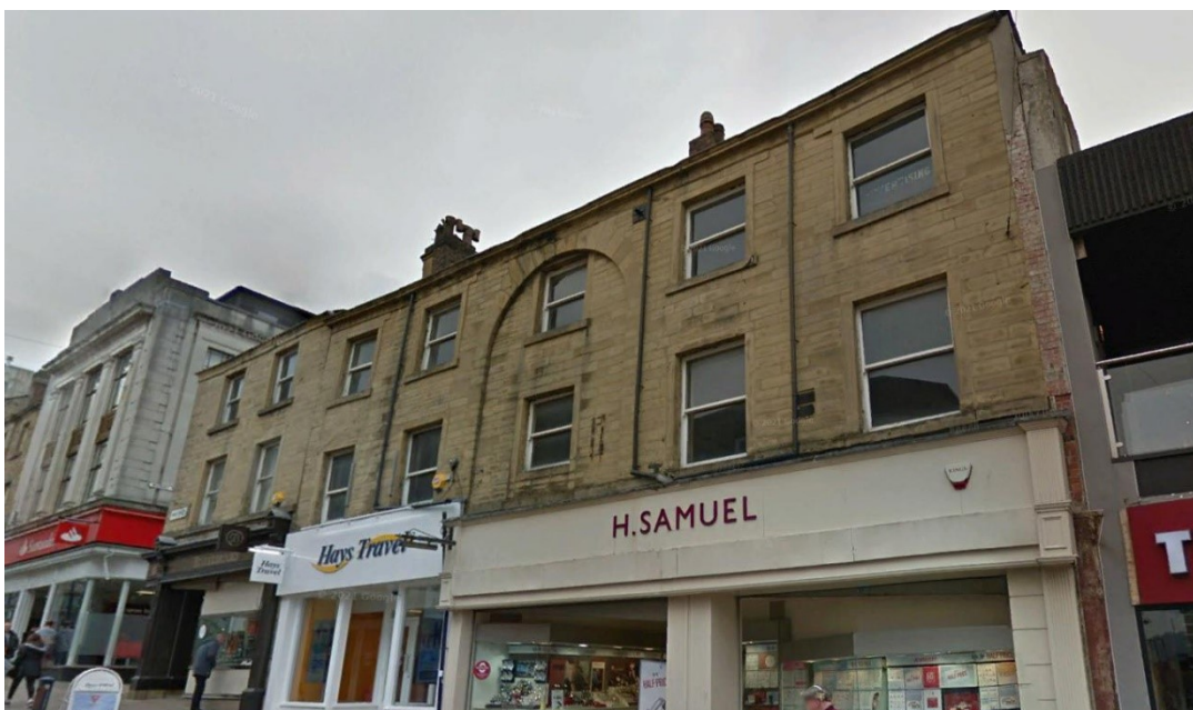
Plate 76 13 King Street & 15 15A and 17, King Street
