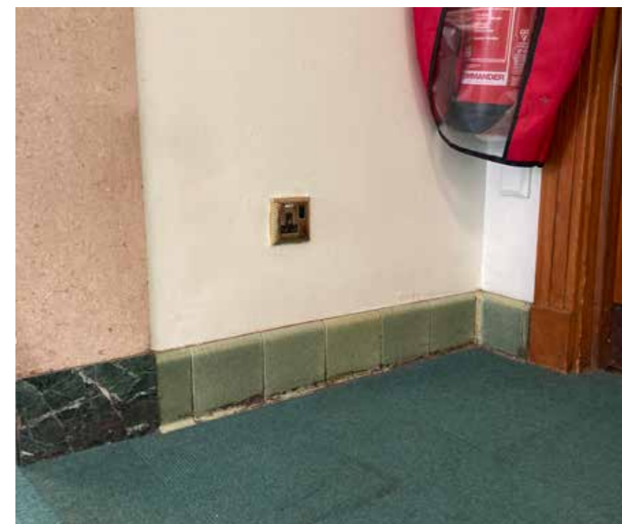
Carpet tiles laid over original / worn floor coverings
