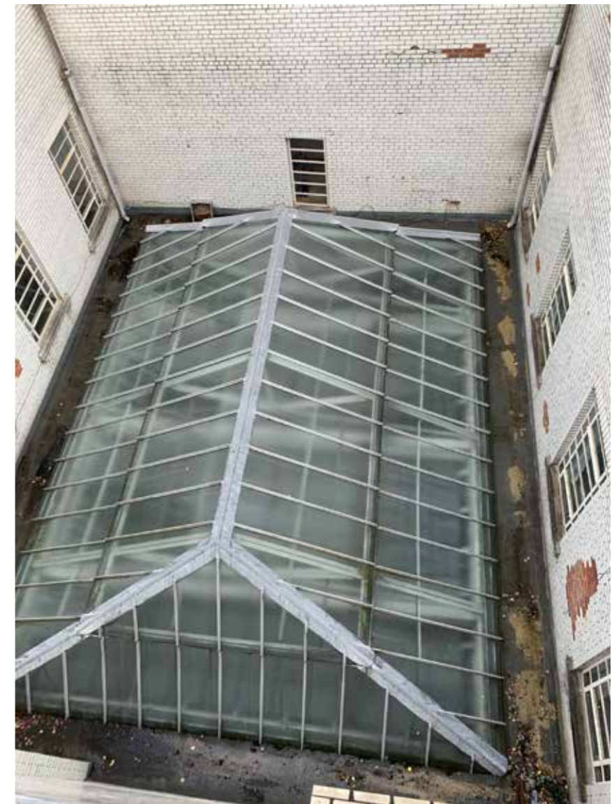
Lantern and north glazed brick wall photographed from roof level
