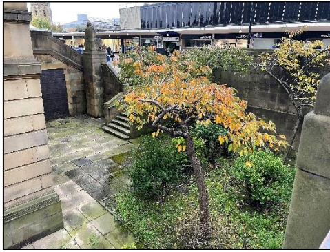
Figure 3 Level difference adjacent to the existing library building
