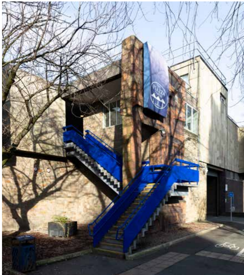
3.5.2.6 - Pedestrian route between Ramsden Street and Queensgate
