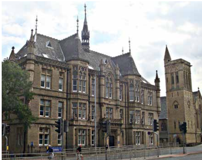
3.5.2.3 - Ramsden Buildings, Queensgate
