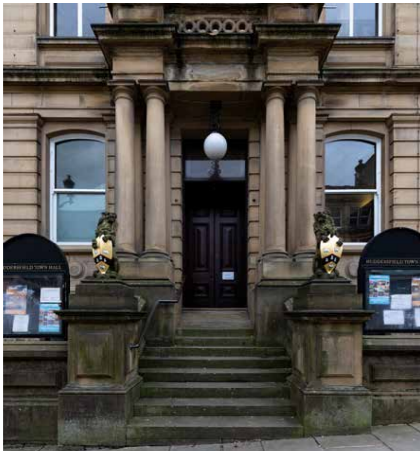
3.7.2.1 - East entrance of the Town Hall, Ramsden Street
