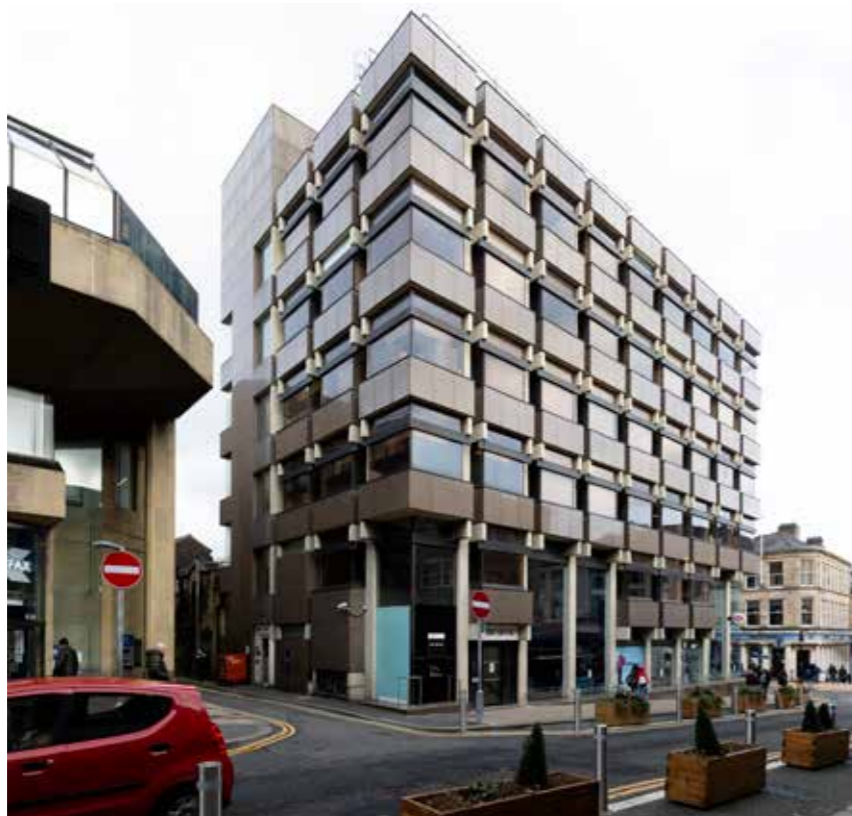
3.1.2.1 - Midland Bank (now HSBC), No.2 Cloth Hall Street
