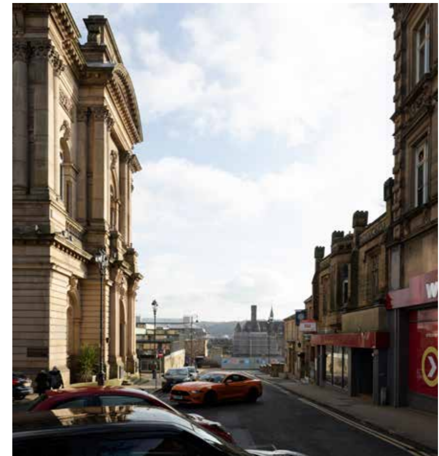
3.6.2.7 - Town Hall (left) and former school building (right) on Princess Street
