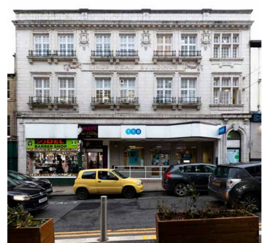
3.1.2.3 - King's Head Buildings, No.19-21 Cloth Hall Street
