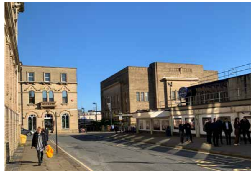
3.7.2.5 - Peel Street looking north
