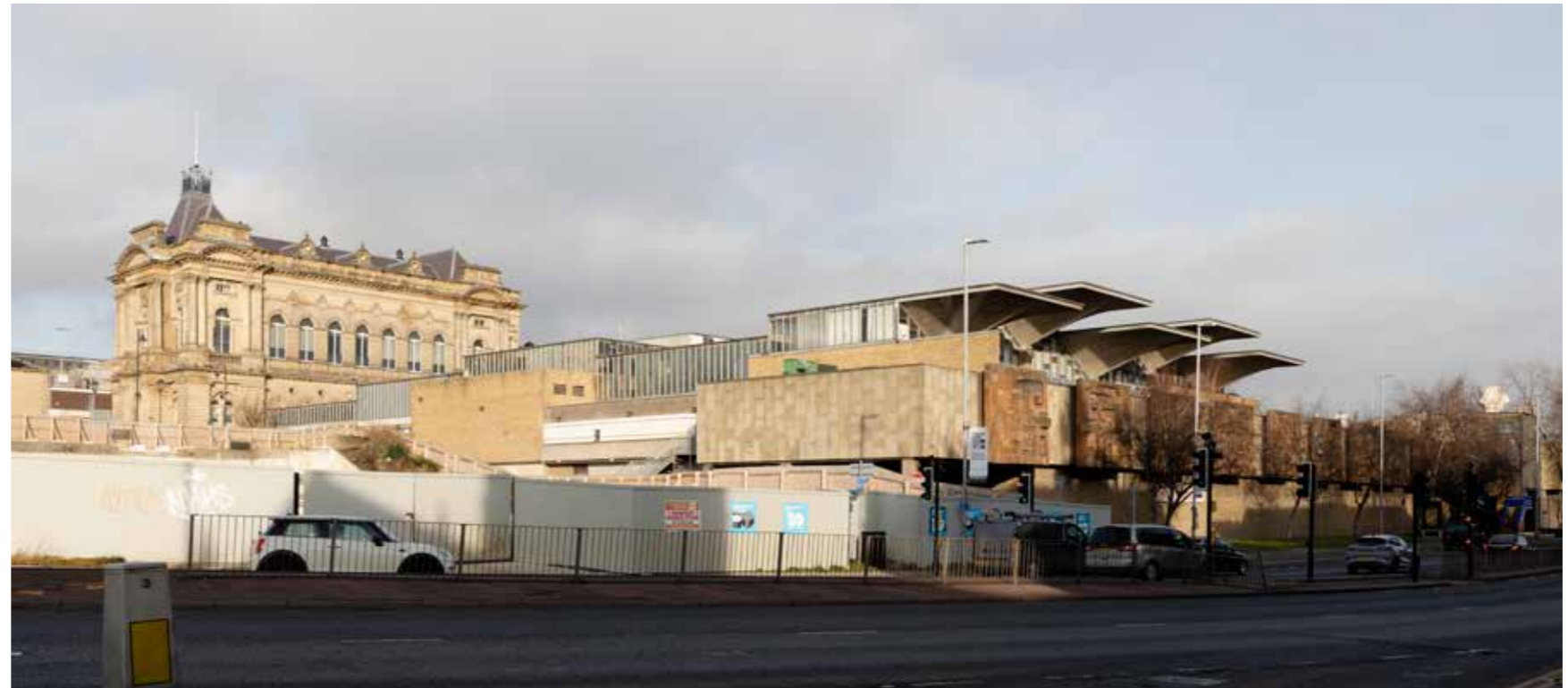
3.5.2.2 - Queensgate at the junction with Queen Street South, looking north-west toward the site
