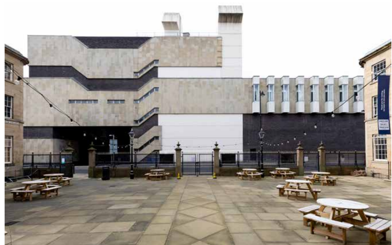
3.3.2.5 - Rear of the Piazza overlooking Queen Street, from the entrance portico of the Lawrence Batley Theatre
