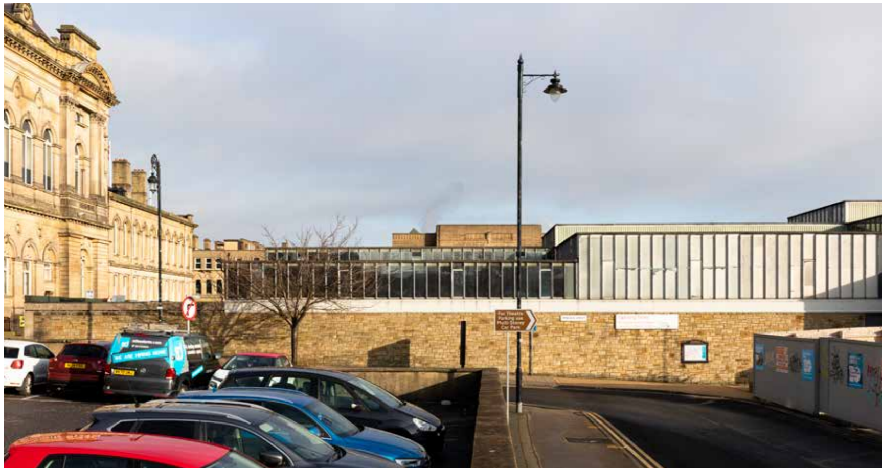
3.6.2.4 - View of south elevation of Market Hall on Princess Street, seen from the car park on Alfred Street
