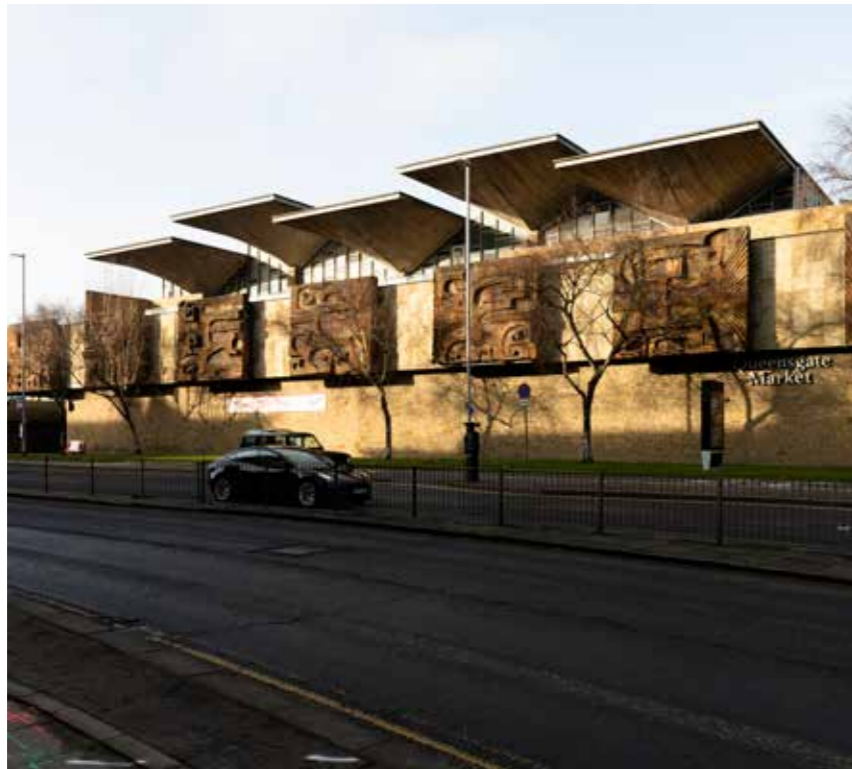
3.5.2.1 - Market Hall, Queensgate
