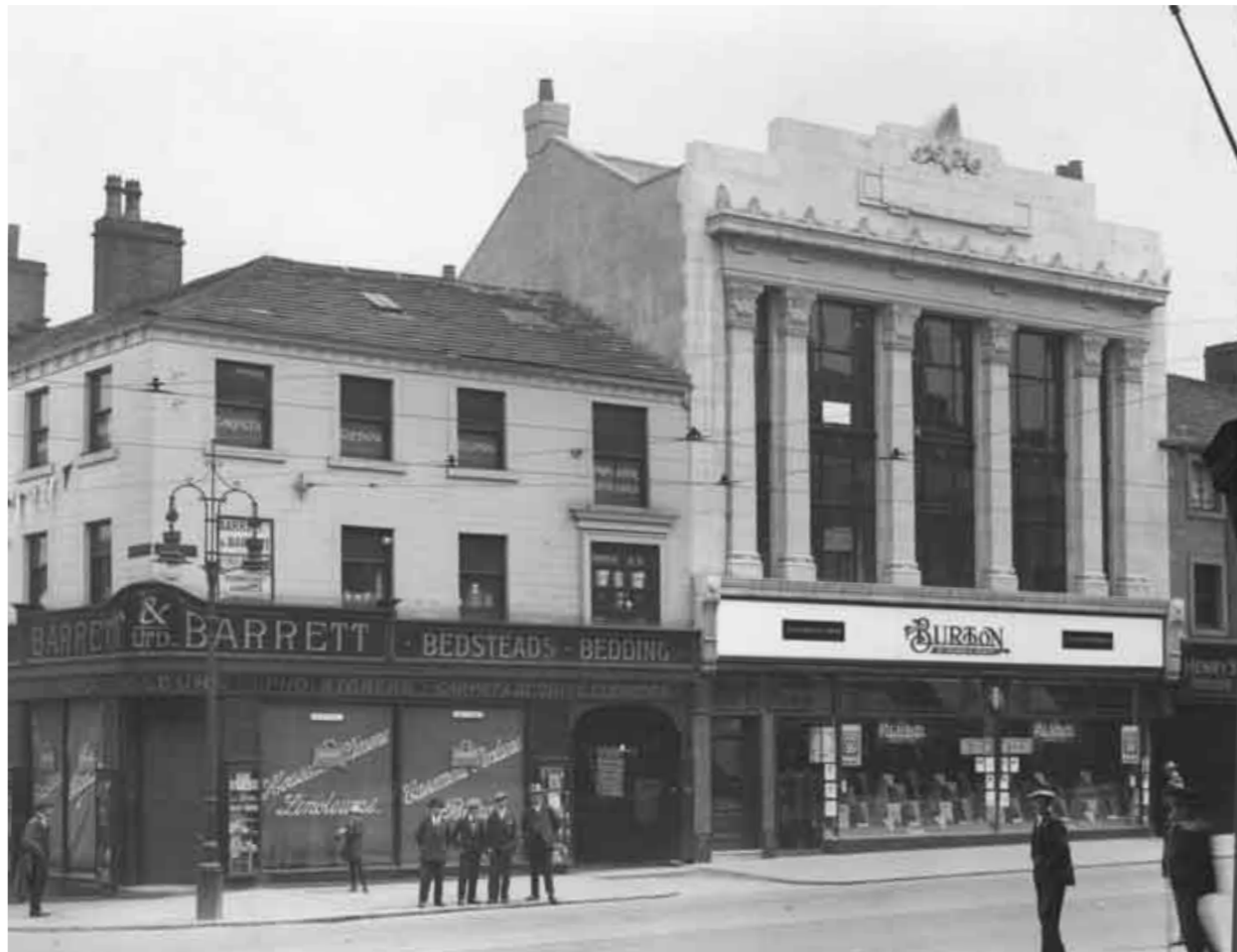
3.1.2.4 - No. 17 and No. 21 New Street (1920s)
