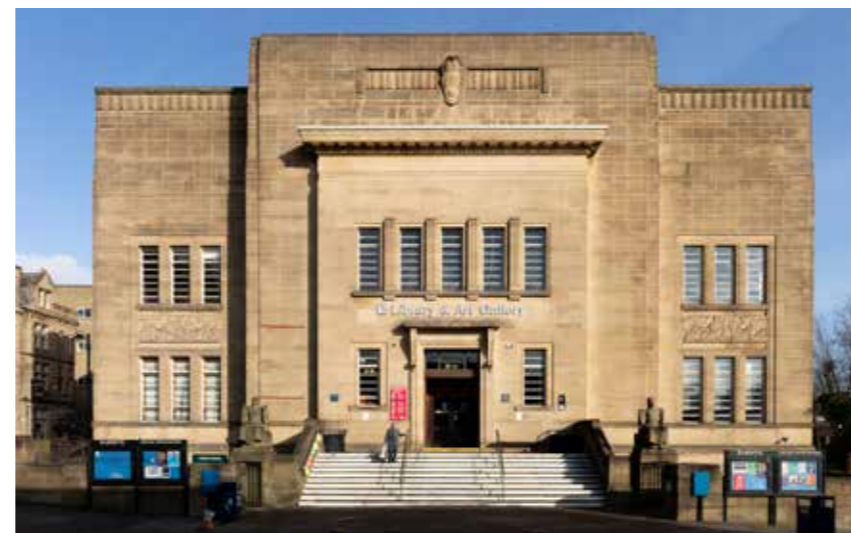
3.8.2.5 - Library and Art Gallery entrance onto Princess Alexandra Walk
