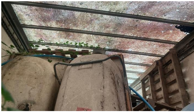
Photo 7: The interior of Building 2, no PRFs visible.
