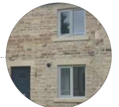
Window head and cill cast stone
