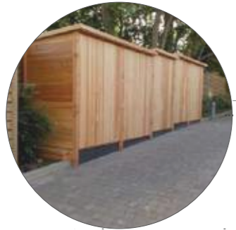
Cycle storage and shared tool sheds with green roof
