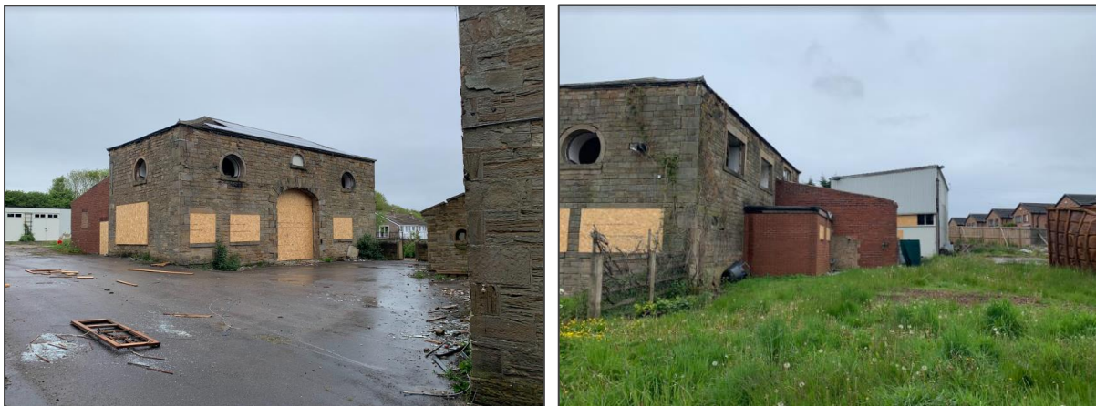
Left Plate 7 – View of south elevation of barn to rear of Clough House from within site to south.
