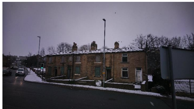
Photo 16-View to front of terrace
