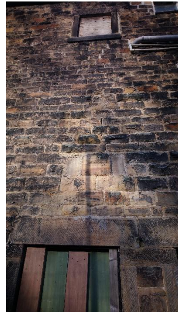
Photo 14-Vertical crack No 4
