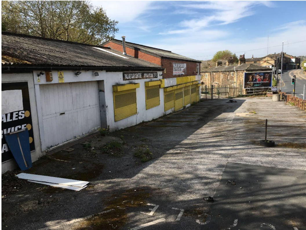
Photo 7. Looking west-south-west along north side of Building 2
