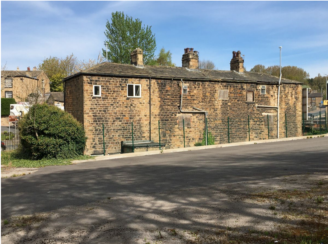
Photo 1. Looking north to rear of terrace houses on the site (Building 1)
