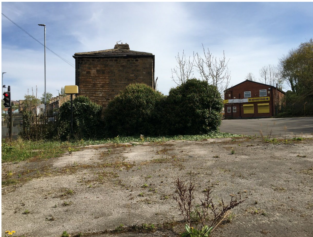
Photo 4. Looking north-east to south gable of terrace houses (Building 1)
