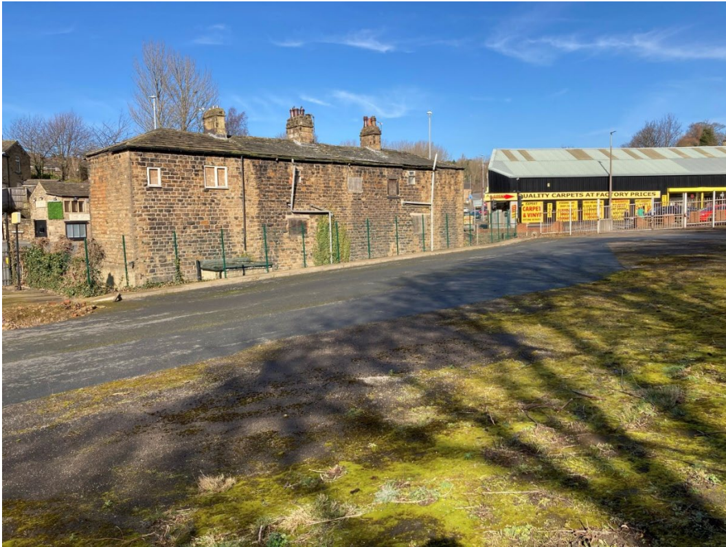
Photo 17. Looking north towards Building 1 (March 2022)
