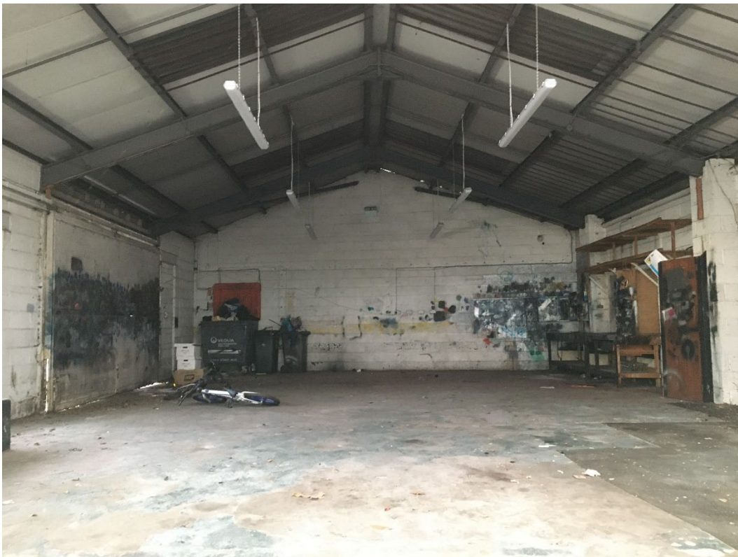
Photo 14. Interior of Building 2
