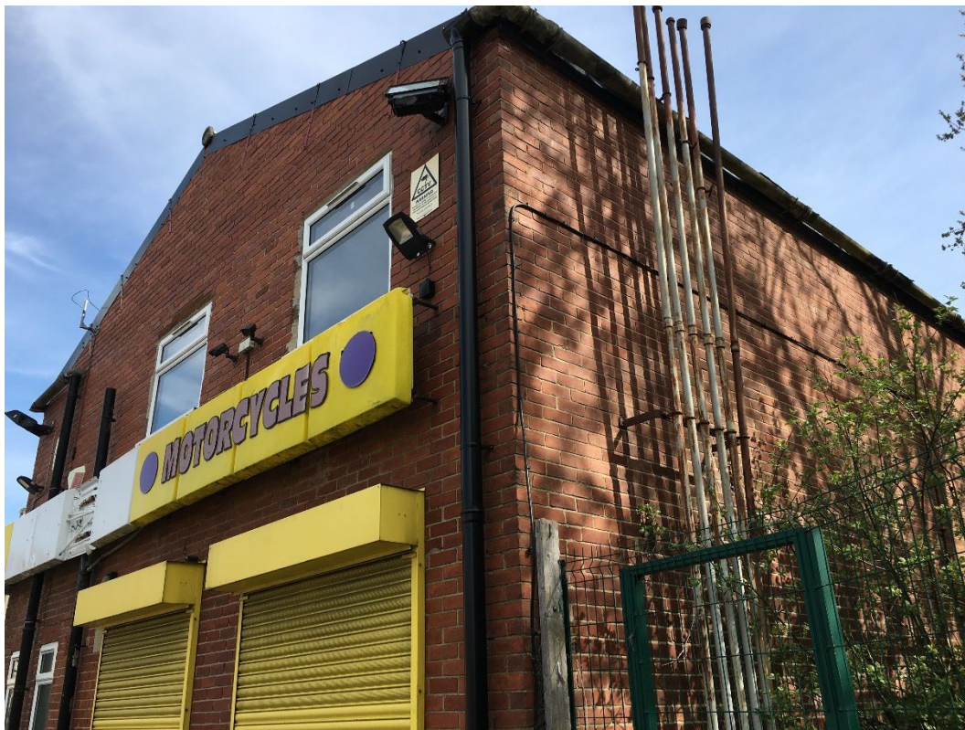
Photo 12. South-west corner of Building 2
