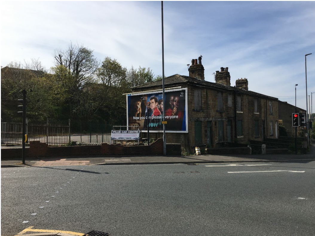
Photo 2. Looking south towards terrace houses (Building 1)
