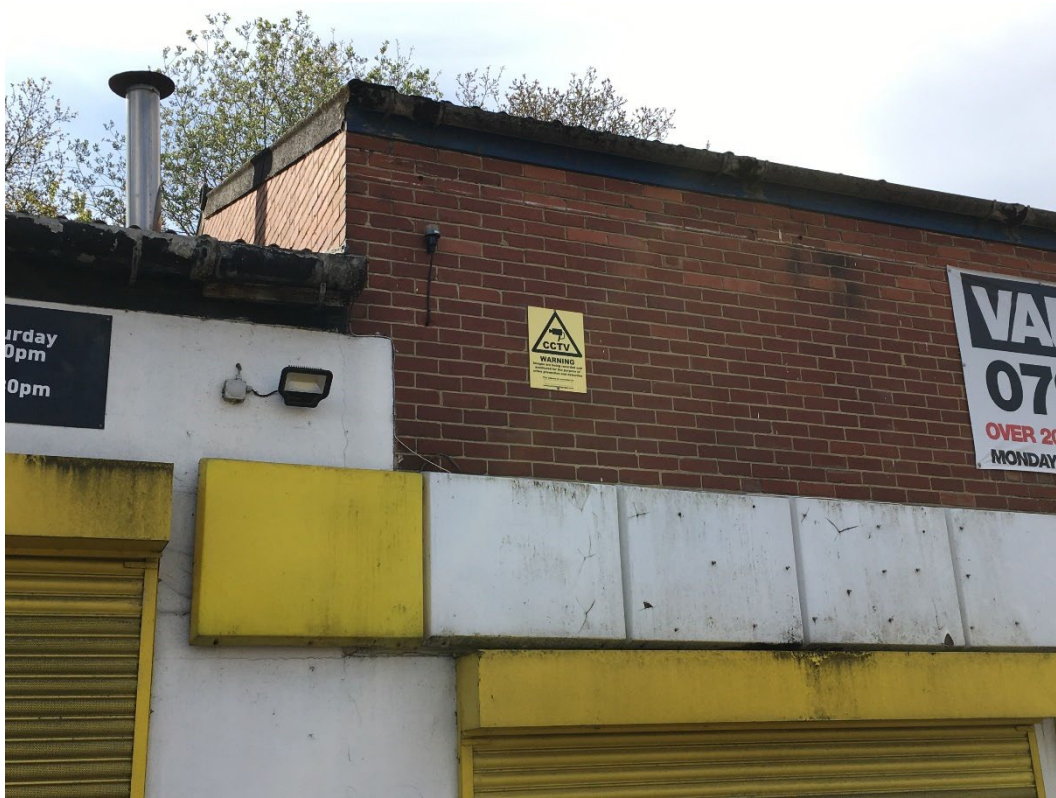
Photo 11. Looking south to Building 2
