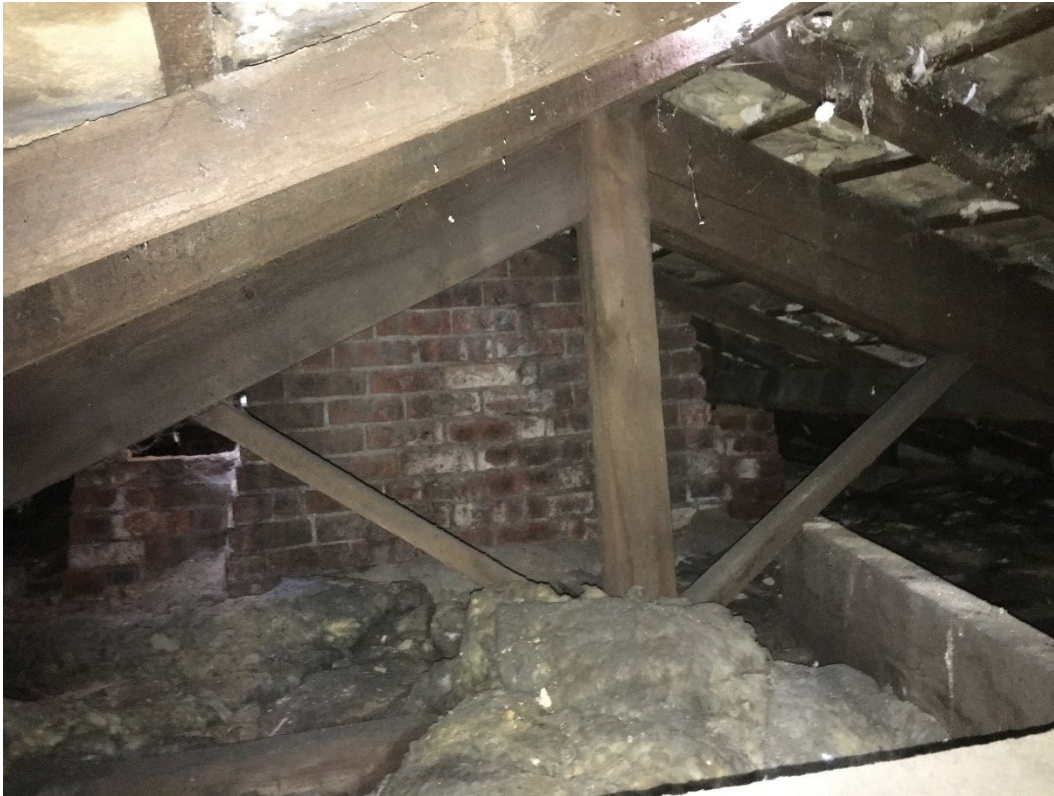
Photo 13. Interior of Building 1 loft space
