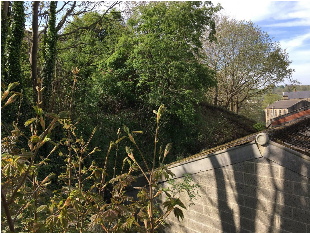
Photo 10. Looking south-west over roof of Building 2
