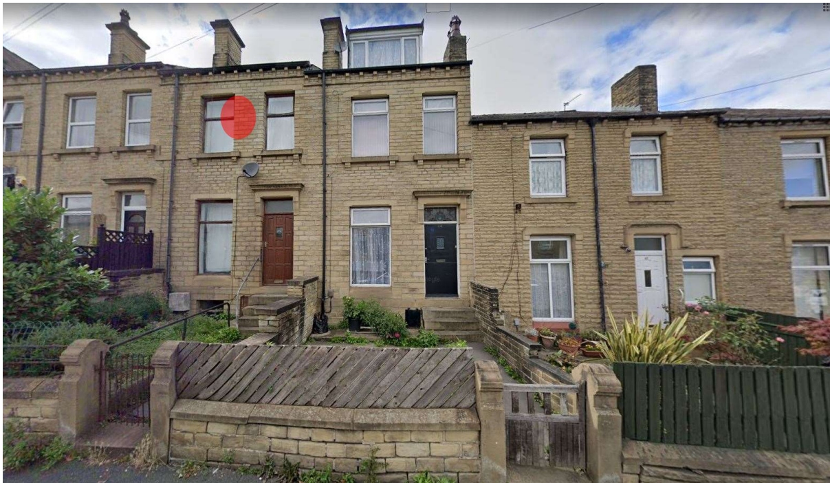
Pic 1- street view of blacker road
