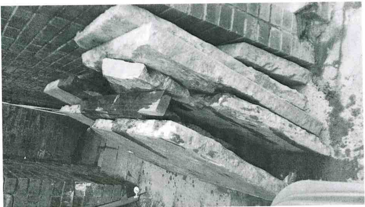
The photograph above shows the Hard York Stone removed from where Hot Tub number 1 sits.
