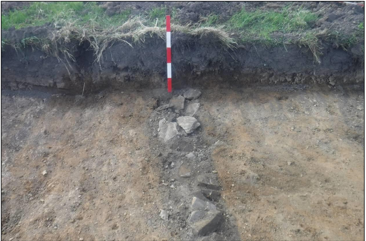
Plate 23. Culvert [1402], looking east.
