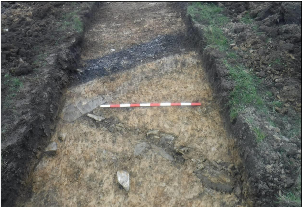
Plate 12. Culvert [802], drain [804] and French drain [806] (pre-ex), looking north.
