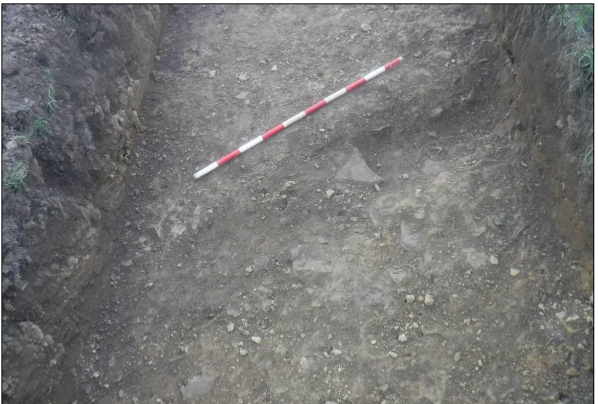
Plate 4. Land drain/culvert [302], looking west.
