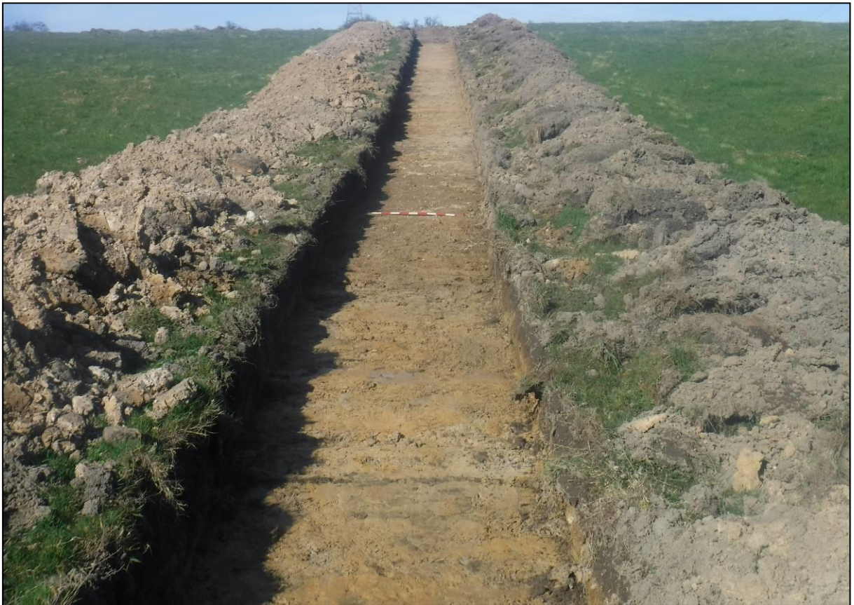
Plate 24. Trench 15, looking west.
