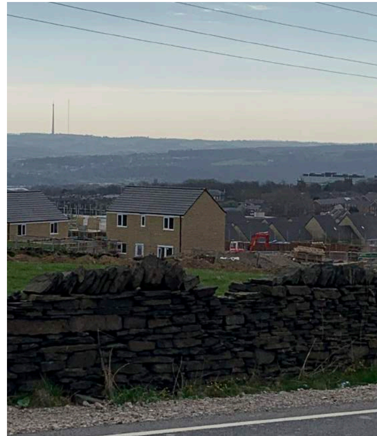
Housing under construction at southern boundary of proposed site
