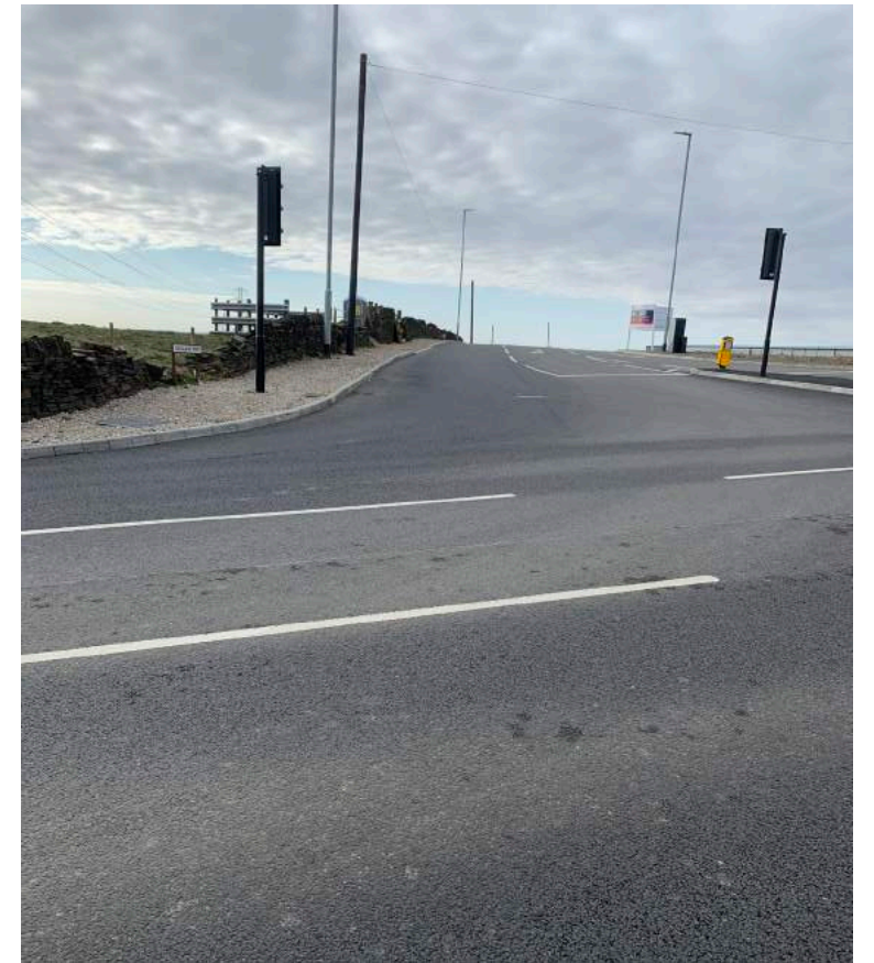
Upgraded road junction of Lindley Moor Road & Crosland Road
