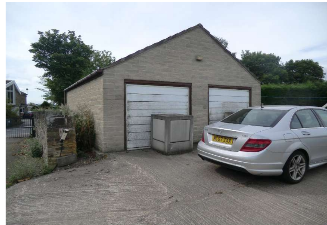
Figure 4 – Existing garage block
