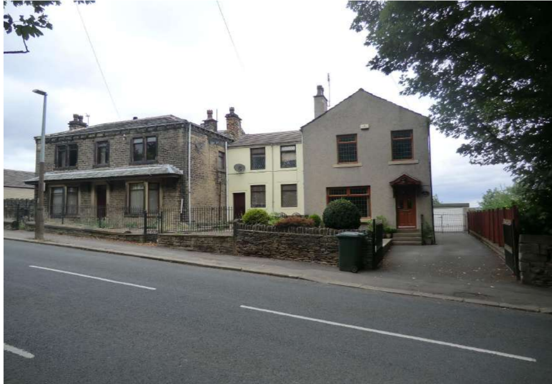
Figure 1 – Existing dwellings as viewed from Whitechapel Road
