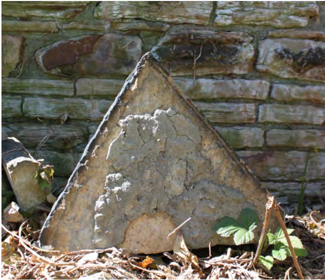
Coping profile, loose on the ground
