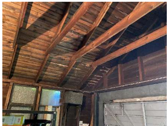
Photograph 8: Interior of Building B1 (07.07.2022).
