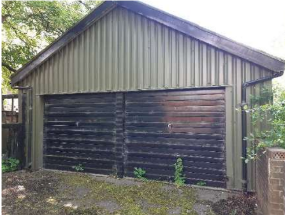
Photograph 5: Building B1, northern aspect (09.06.2022).
