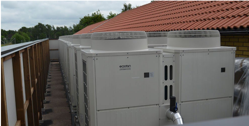
Figure 5: Typical Centralised ASHP Cascade within External Enclosure
