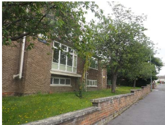
Existing building along Hurst Knowl
