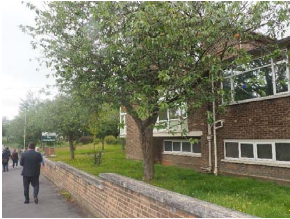
Existing building along Hirst Knowl
