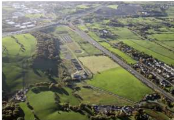
Figure 2: Aerial photograph of the site, looking southwards the M62 Chainbar roundabout
