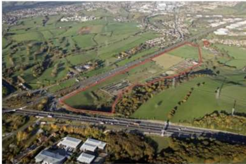
Figure 3.2: Aerial Photograph of the Application Site Outlined in Red
