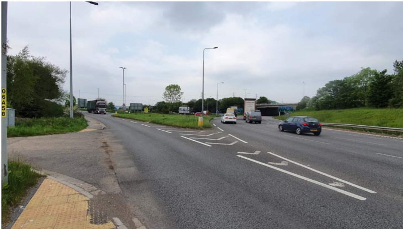
Photo P4 View looking north towards the proposal site from Chain Bar roundabout J26 of the M62/M606 interchange. The proposal site is located beyond the elevated section of motorway in the centre of the photograph.
