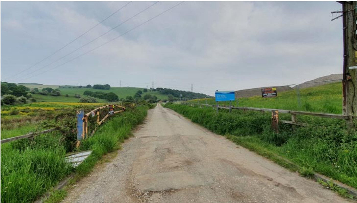
Photo P5 Photograph looking south along the existing access to the waste water treatment plant and the proposal site is located beyond and beneath the electricity cables in the distance.
