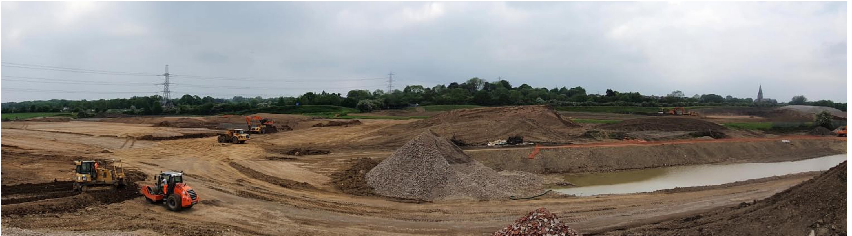
Photo P2 View looking west across engineering works. The proposal site is located beyond the left of the photograph. The view is from a temporary elevated location on a spoil mound.
