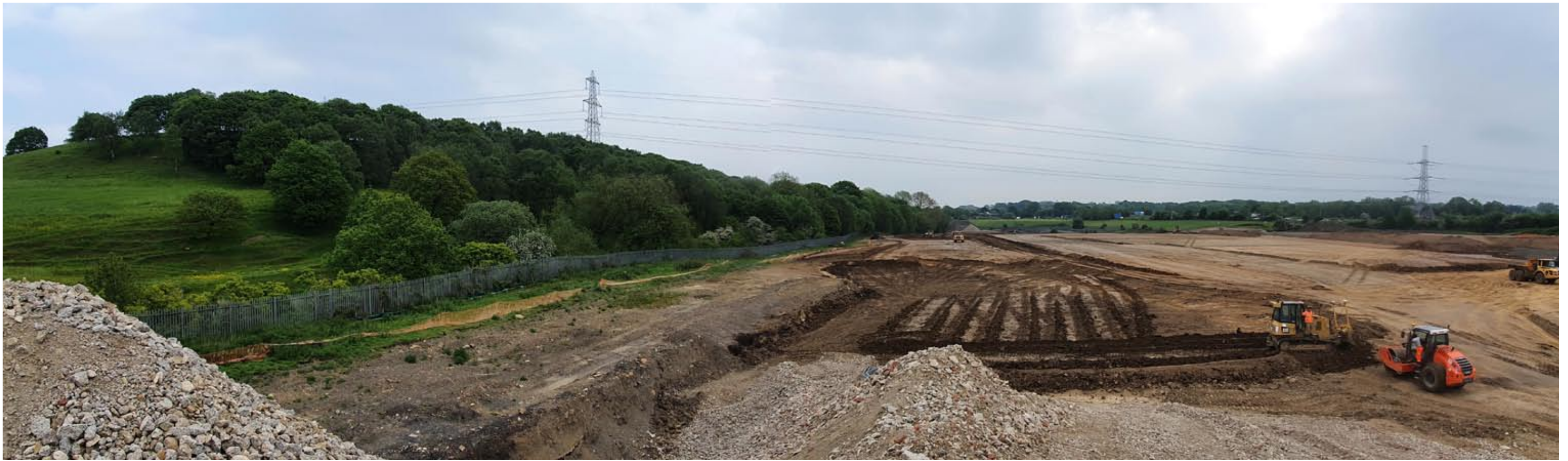
Photo P1 View looking south across engineering and regrading works to the approved development site. The proposal site is located beneath the overhead electricity cables to the rear of the photograph. The view is from a temporary elevated location on a spoil mound.
