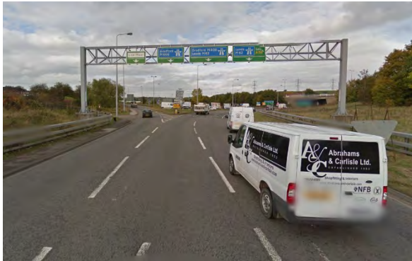
1) Roundabout at junction of M62 / M606 looking towards Bradford Road
