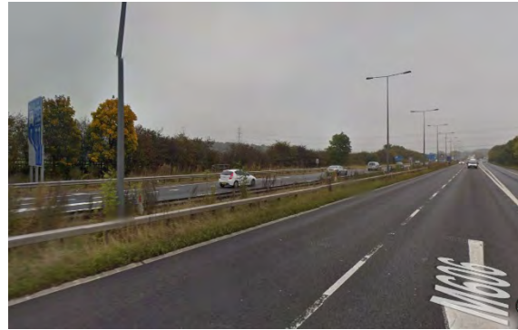
2) View south along M606 showing existing landscaping to western boundary of the proposed site
