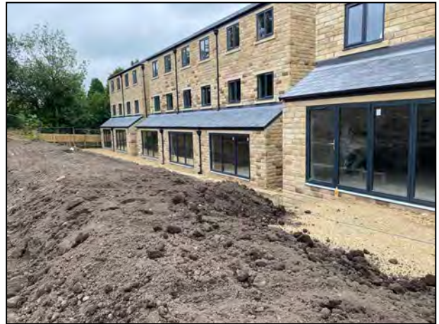
View over the newly laid 600mm thick topsoil in rear gardens of 7 – 13 house plots
