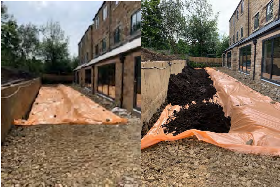
Figure 5 Geotextile and first layer of topsoil laid in lower rear gardens
