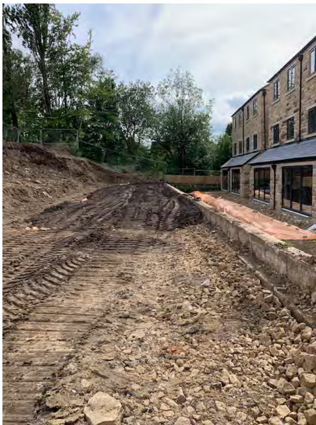
Figure 5 Geotextile and first layer of topsoil laid in upper rear gardens
