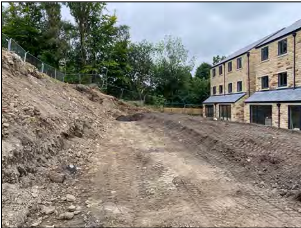
View over the newly laid 600mm thick topsoil in rear gardens of 7 – 13 house plots
