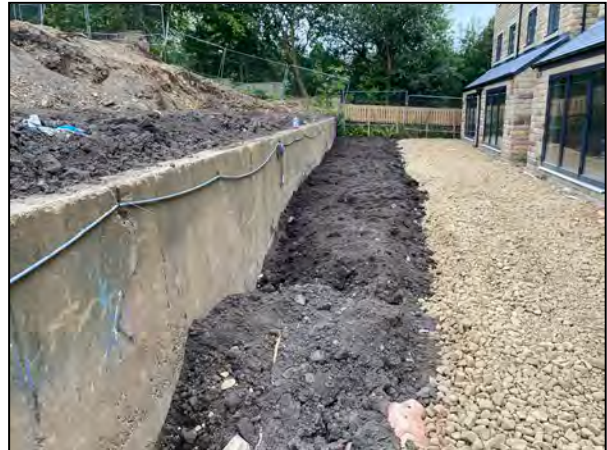
View along retaining wall showing topsoil on upper and lower garden levels where trial pits were excavated. Aggregate laid over geotextile shows areas where hard cover will be laid.
