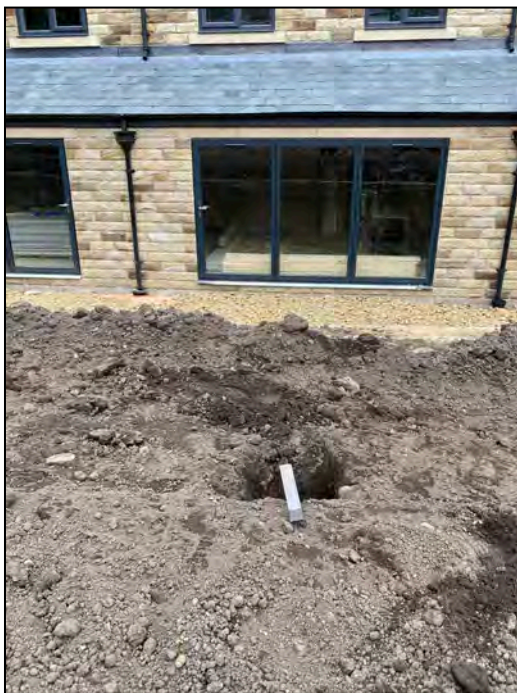
Trial Pits outside House Plot No 9 confirming 600mm of topsoil
