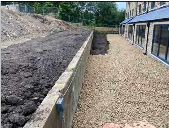
View along retaining wall showing topsoil on upper and lower garden levels where trial pits were excavated. Aggregate laid over geotextile shows areas where hard cover will be laid.
