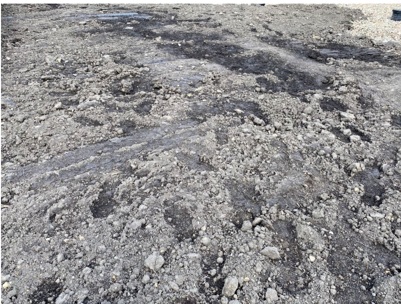
Detailed view of clean topsoil laid
