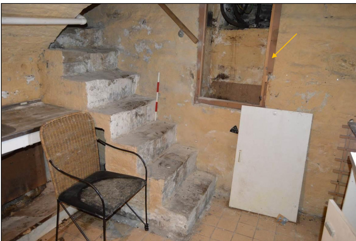
Photograph 16: Stone steps to cellar with former window splay indicated to north elevation (facing north). Scale 0.5m.
