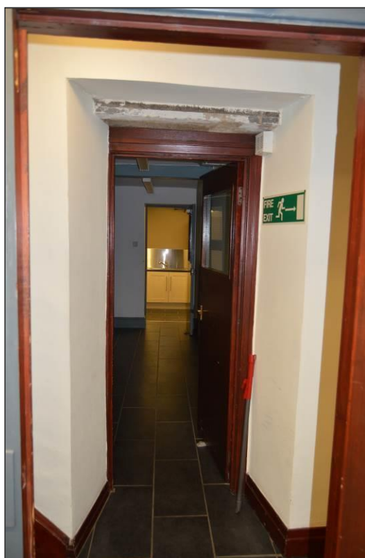
Photograph 24: Internal link through north elevation of three storey weaver's house to later extensions.
