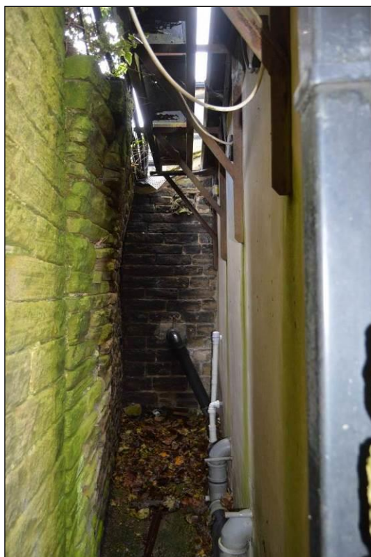
Photograph 36: East elevation to Building 3.
