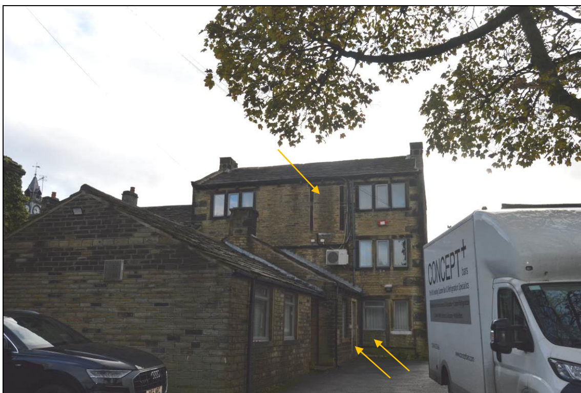
Photograph 13: Rear aspect of Midway house (facing south), with its series of extensions to foreground. Historic, blocked doorway apertures are indicated.
