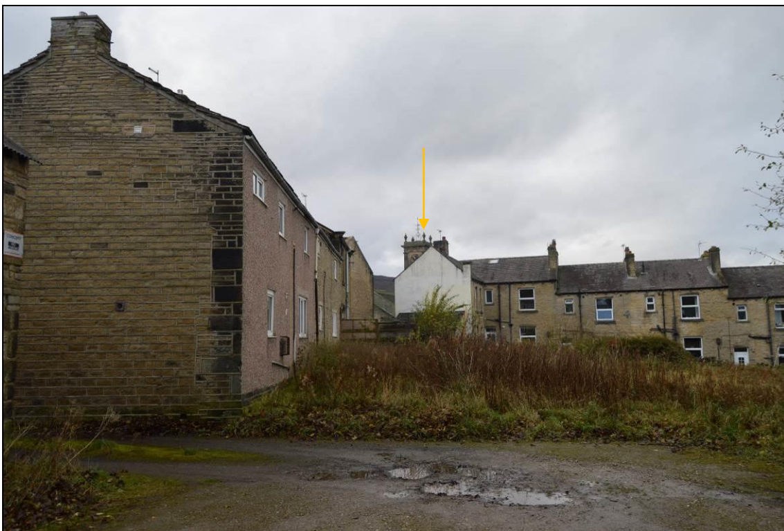
Photograph 7: Rear aspect of the undeveloped portion of the Midway House property (facing west). Beyond the terrace backs is the tower of St Bartholomew's Church.
