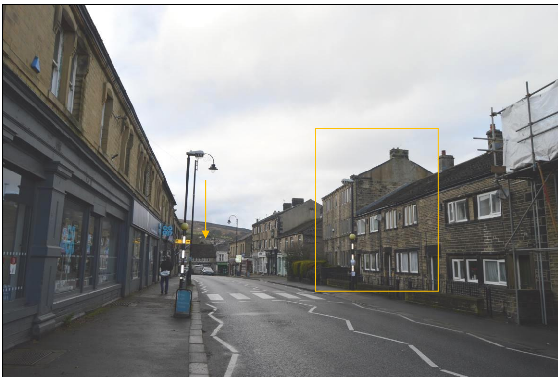
Photograph 1: Huddersfield Road approaching from the east towards the Market Place (looking north west, with Wessenden Head in the background) with the Midway House (Building 1, also indicated).
