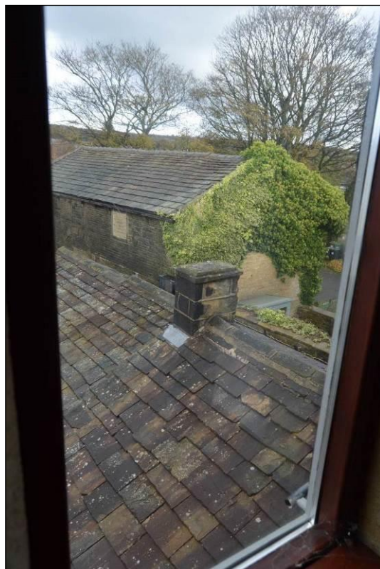
Photograph 32: Capped chimney stack of building 2.
