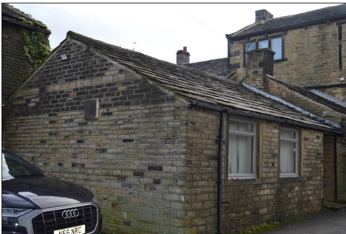
Photograph 35: Exterior to building 3.
