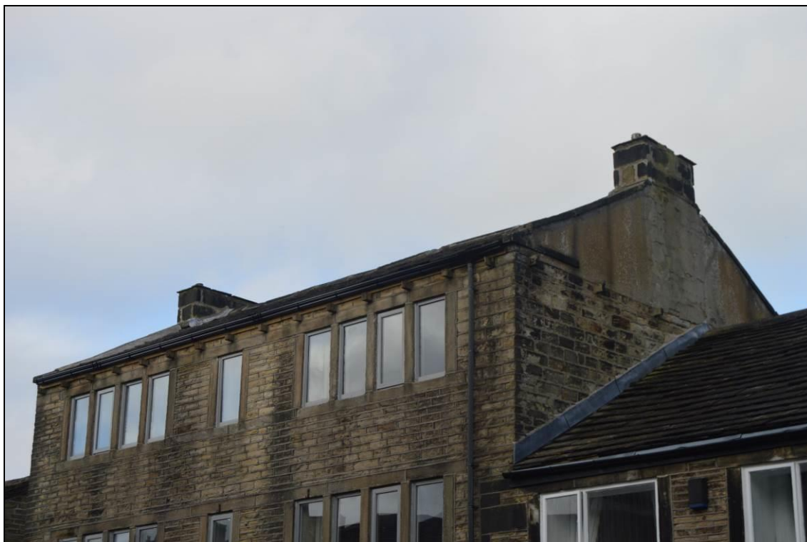
Photograph 11: Stone corbels set below the roof line and east gable features (facing north west).
