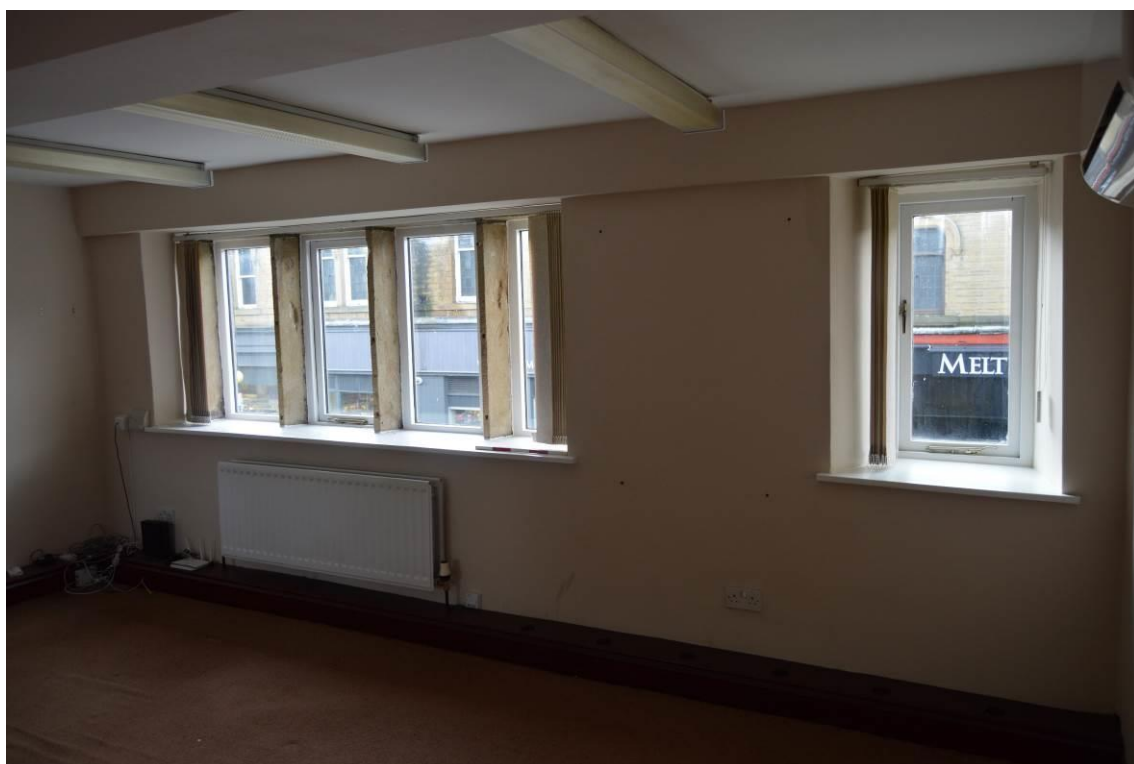
Photograph 28: First floor room front aspect. Scale 0.5m.
