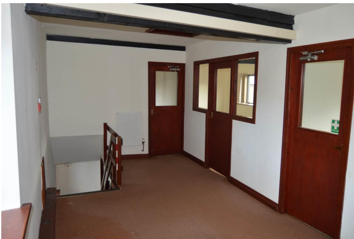
Photograph 29: Second floor landing. Scale 0.5m.
