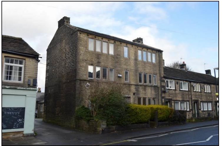
View of Midway House from Huddersfield Road, Meltham
