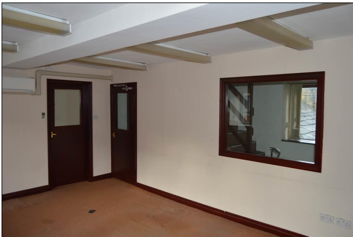
Photograph 27: First floor partitioned room. Scale 0.5m.
