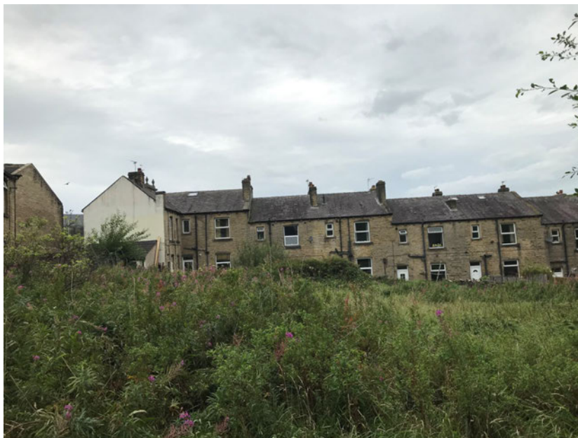
Image 4 - Terrace properties to West of site.
