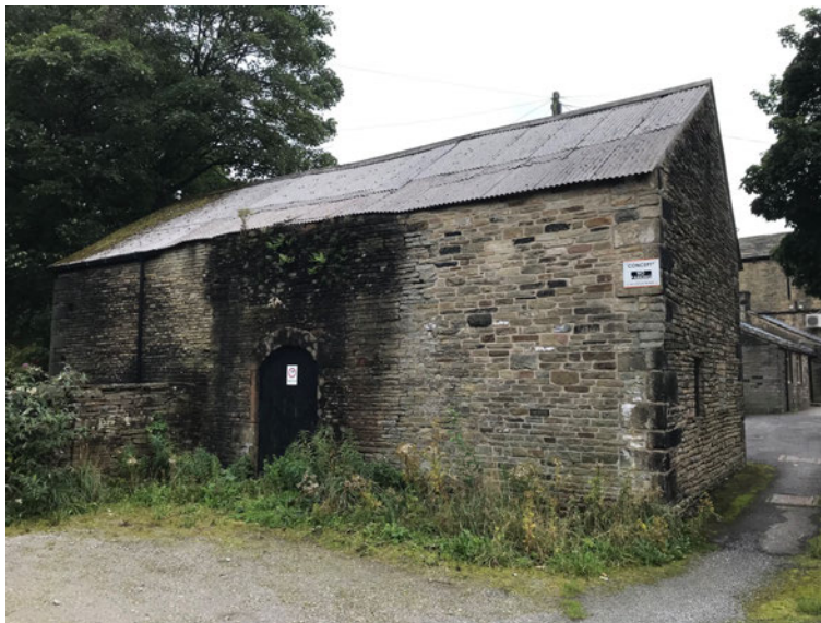
Images 6 and 7 - Outbuilding to be demolished
