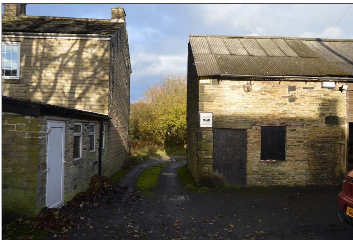
Photograph 5: Present access to the rear areas of the property's plot (looking north).
