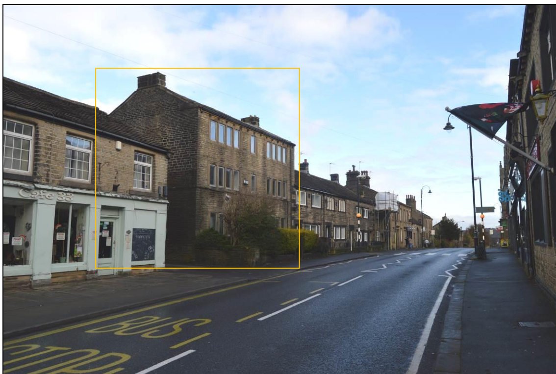
Photograph 2: Huddersfield Road approaching along from the west (looking north east) east towards the Market Place (looking north west) with the Midway House (building 1, indicated).
