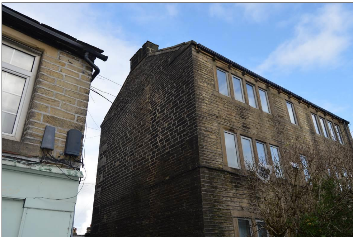
Photograph 12: West gable of Midway House (facing north east).
