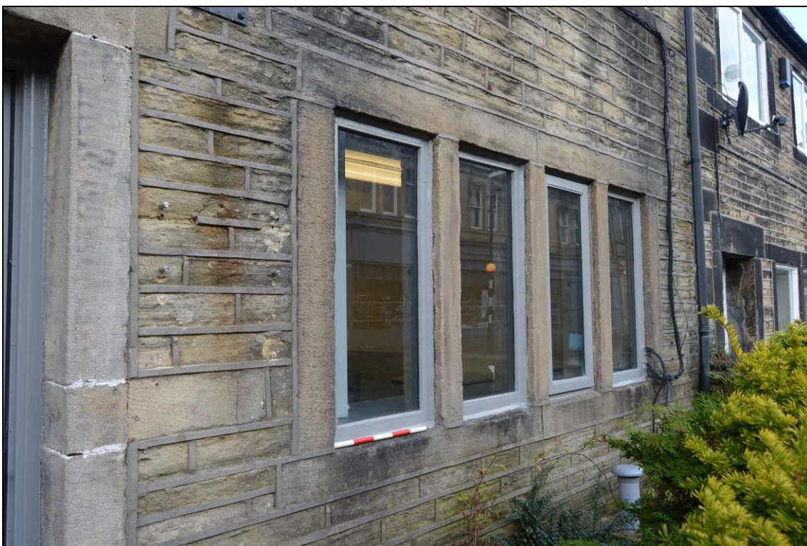
Photograph 9: Example of stone mullion windows to south elevation, ground level (facing north east). Scale 0.5m.
