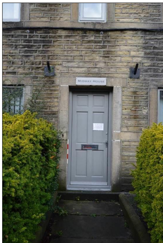
Photograph 10: Front door (facing north). Scale 0.5m.
