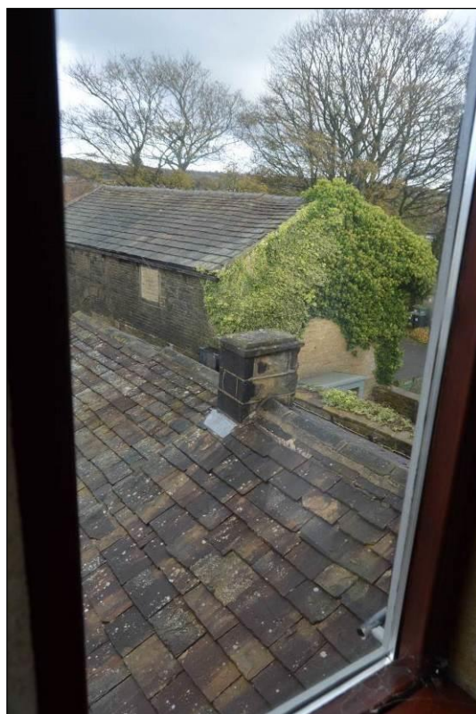
Photograph 32: Capped chimney stack of building 2.
