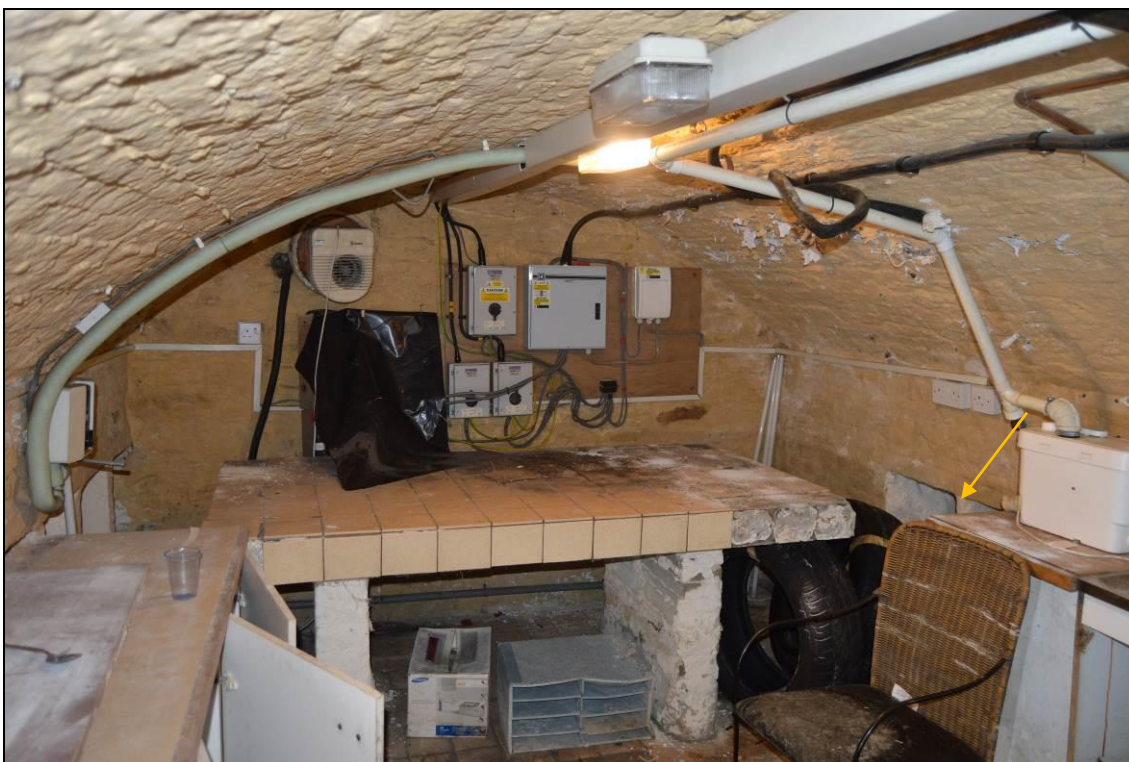
Photograph 18: The barrel vaulted cellar of the Midway House (looking south). Example of stone furniture indicated.
