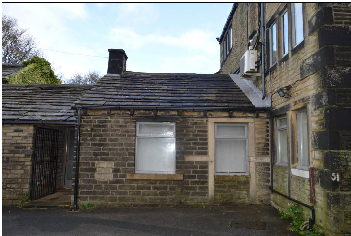
Photograph 31: West facing elevation of single storey extension (building 2). Scale 0.5m.
