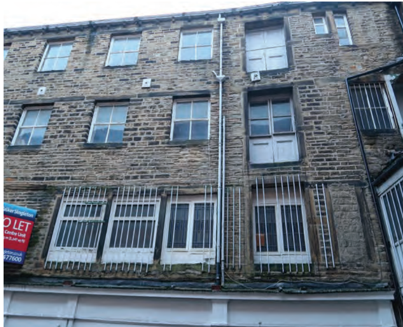
External images of the rear mill range along Albert Yard. Note the lower floors where the potential of infilled Mullions are present indicating that the rear lower storey potentially has older origins with the upper floors being later additions.
