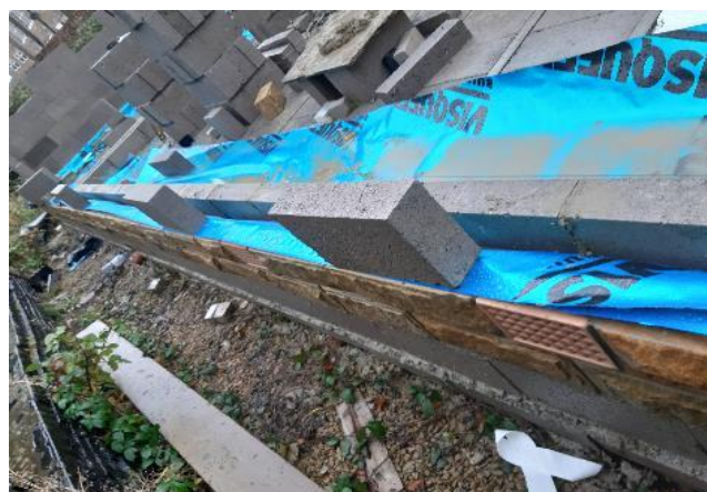
Details of gas membrane during installation; crossing the cavity at the external walls and continuous beneath internal walls.
