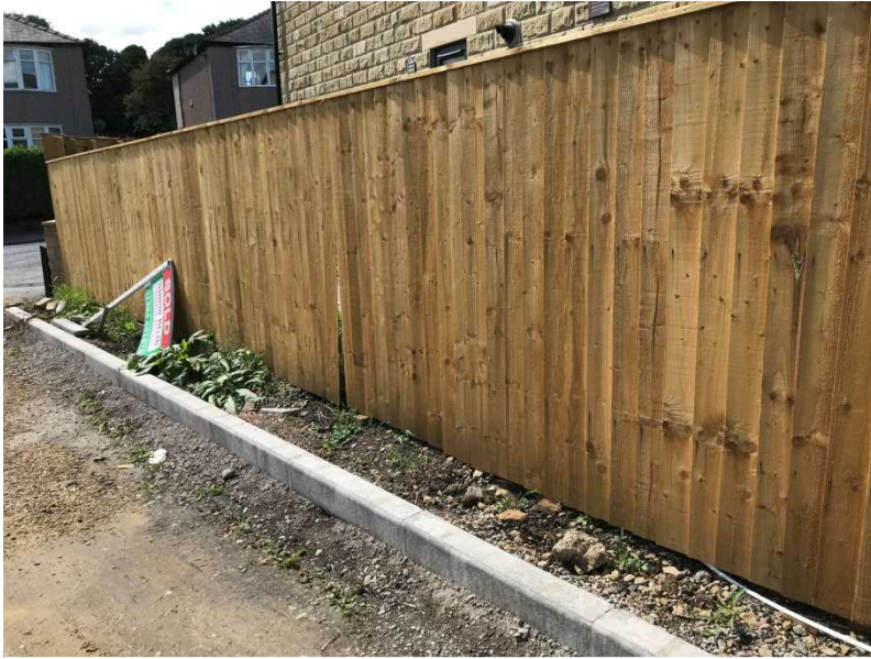
Image 4 - Close Boarded Timber Fence
