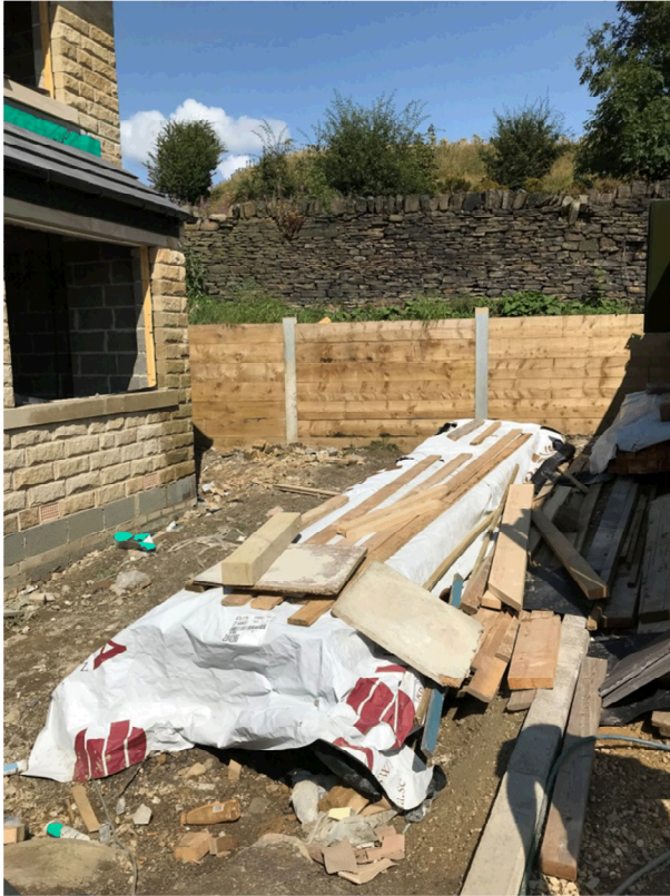
Image 2 - Timber Sleeper Retainer to Existing Drystone Wall
