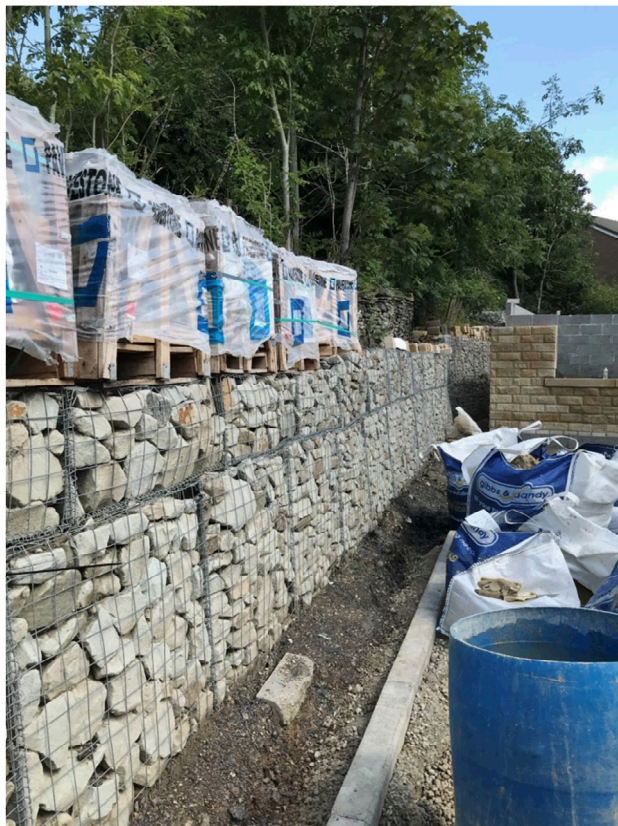
Image 3 - Stone Gabion Retainer to Existing Drystone Wall
