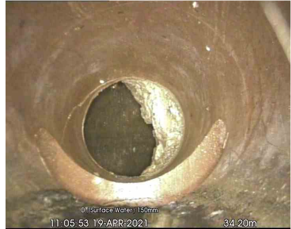
SW1-SW2_34-20m_110553.jpg, 00:07:40, 34.20 m General remark, DROP SHAFT
