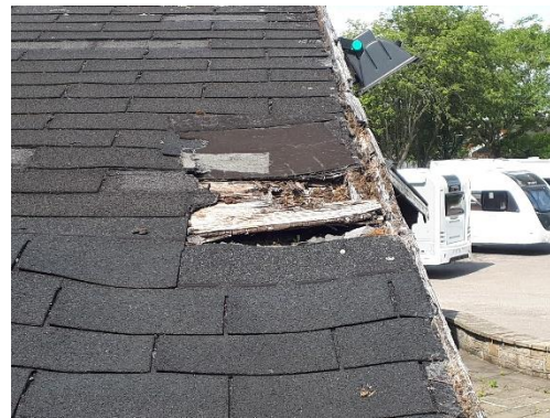
Image 15: Close up of potential roost feature (B1)
