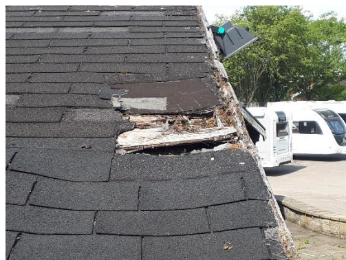
Image 15: Close up of potential roost feature (B1)
