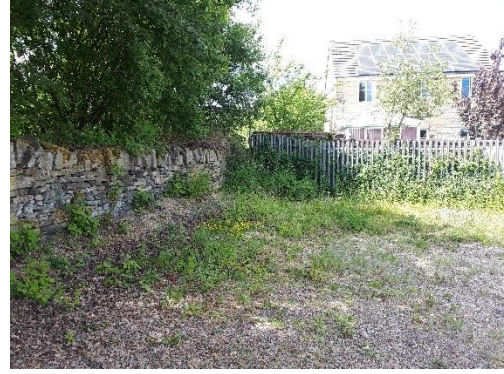
Image 07: Example of bare ground with colonising vegetation (TN6)
